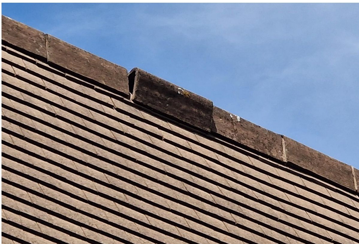
Plate 14: image showing the ridge vent on B1 .
