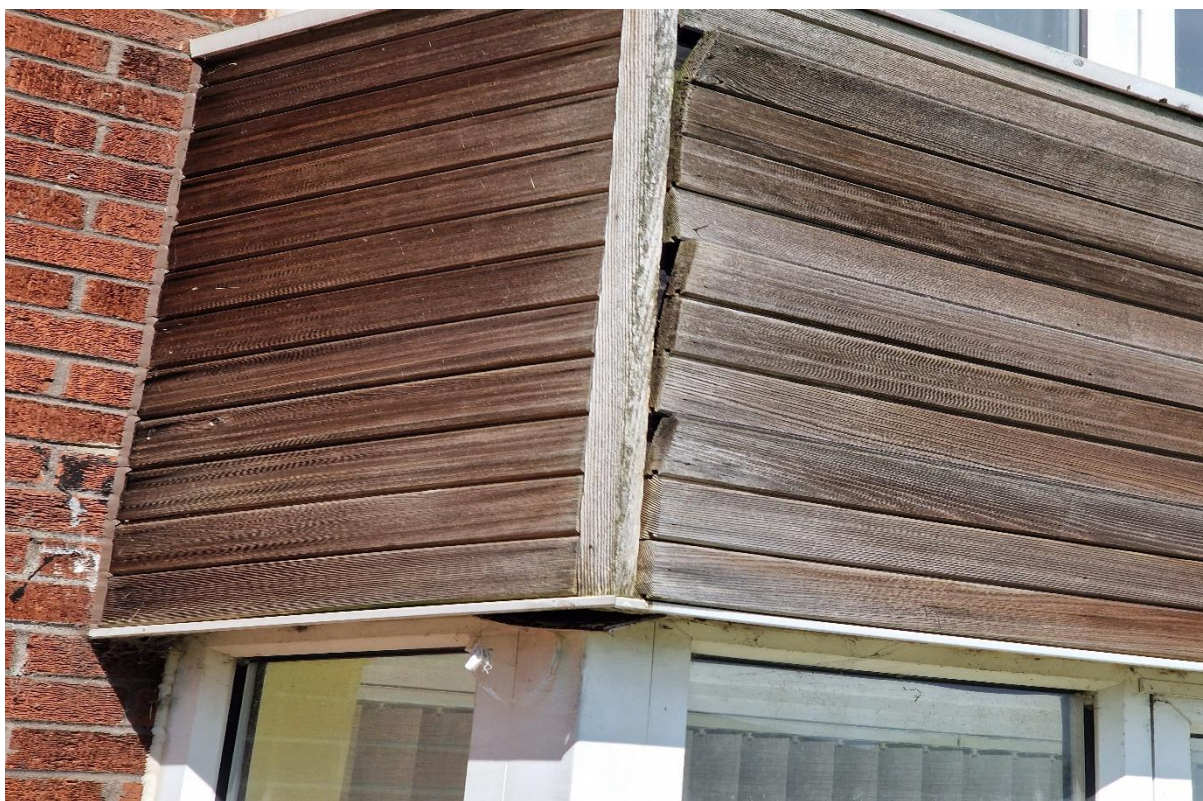
Plate 16: Image showing the missing wood panels on B3 .
