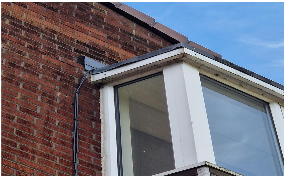
Plate 12: Image showing the missing edge tile on B1 .
