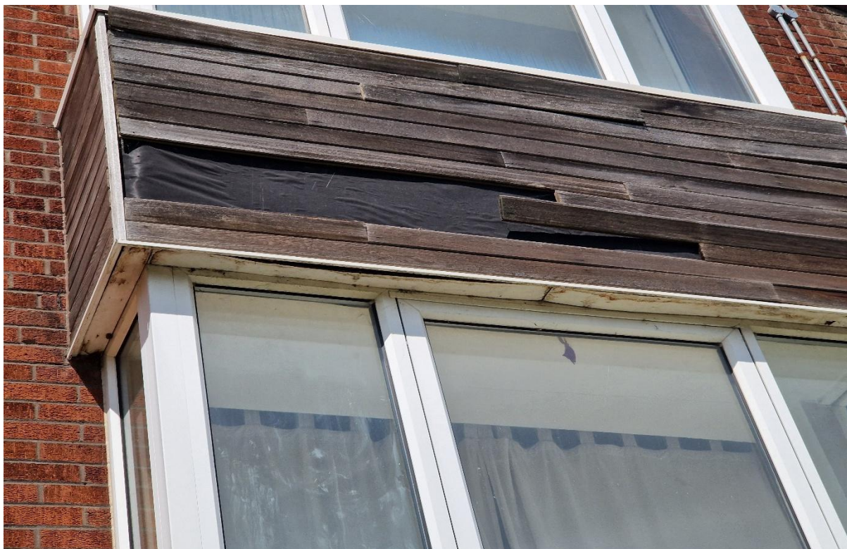
Plate 16: Image showing the missing wood panels on B3 .
