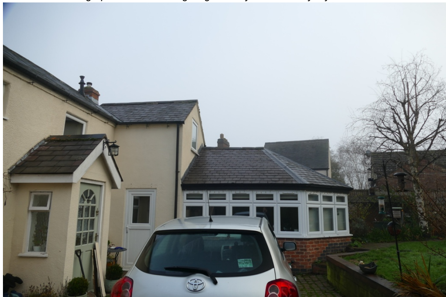
Photograph 3 – the dwelling single-storey conservatory-style extension.
