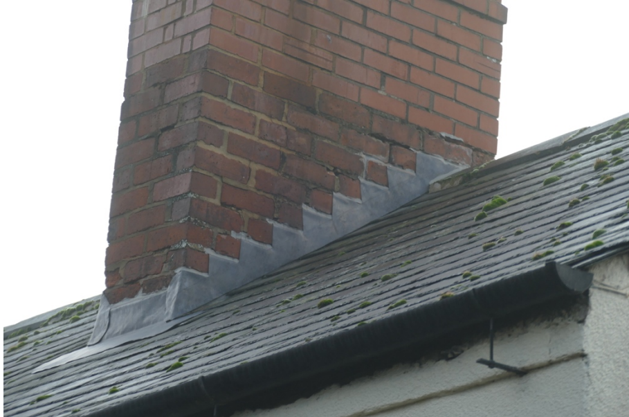
Photograph 5 – recently replaced leading detail.
