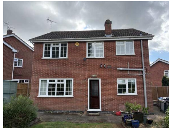
Building B1 – northern (rear) elevation
