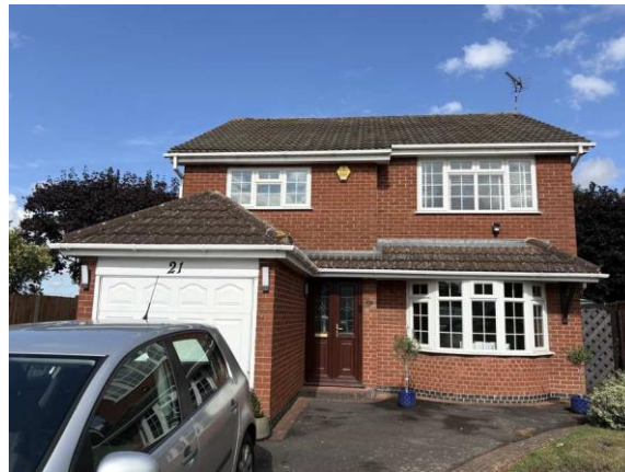
Building B1- southern (front) elevation
