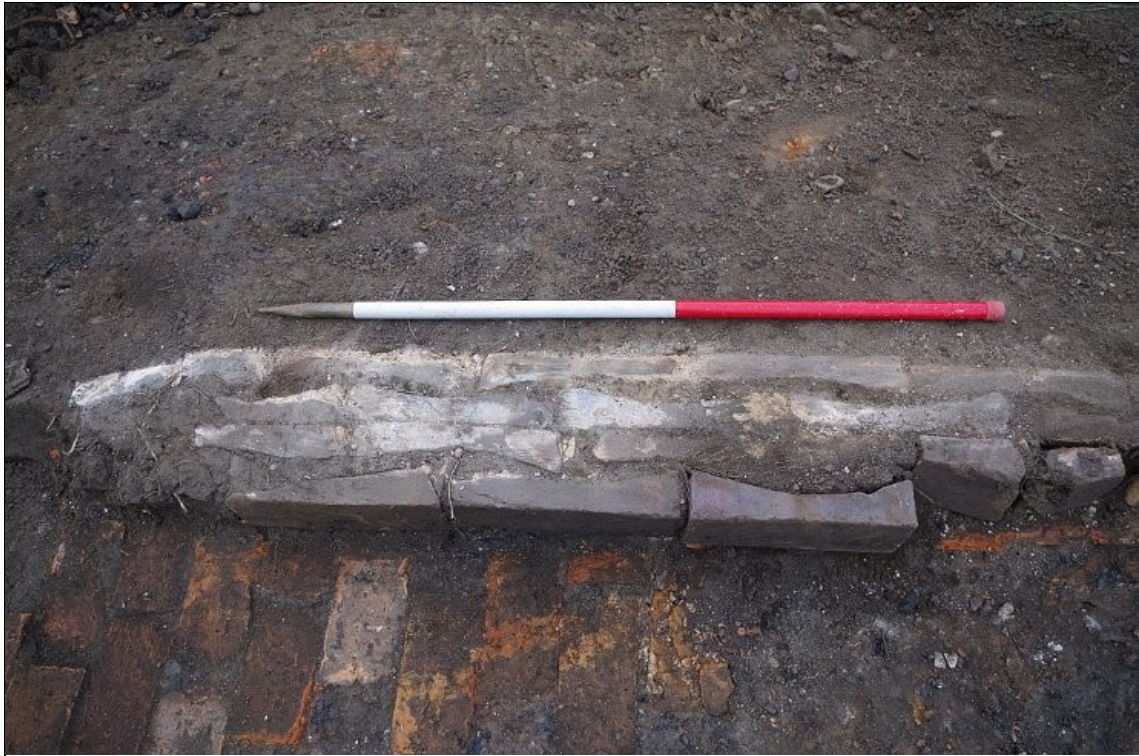
Photo 23. Part of north wall foundation of Area B building composed of reused drainage bricks [29] and internal floor surface [34], looking WNW.
