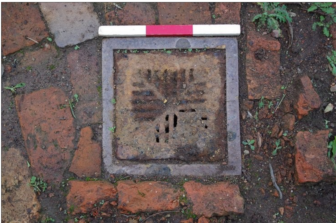
Photo 24. Drainage gully with iron grid [39] set into external surface [11] outside SW corner of Area B building, looking N.
