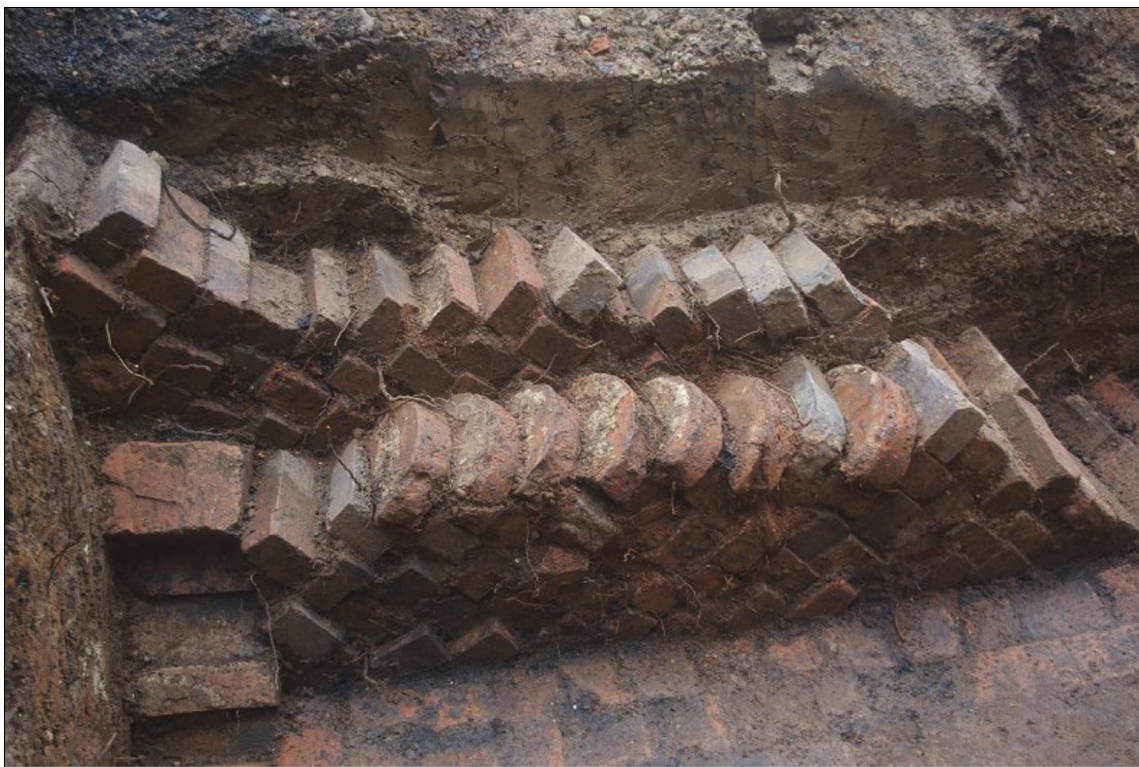
Photo 16. Detail showing reused saddleback coping bricks in retaining wall [03], looking N.
