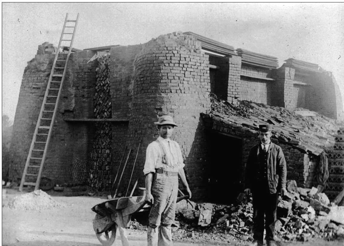
Figure 14. Scotch Kiln at Bottesford, Leicestershire in 1910. Note wicket closed with bricks laid in herringbone fashion and lean-to structure along side of kiln. Bottesford History Group.
