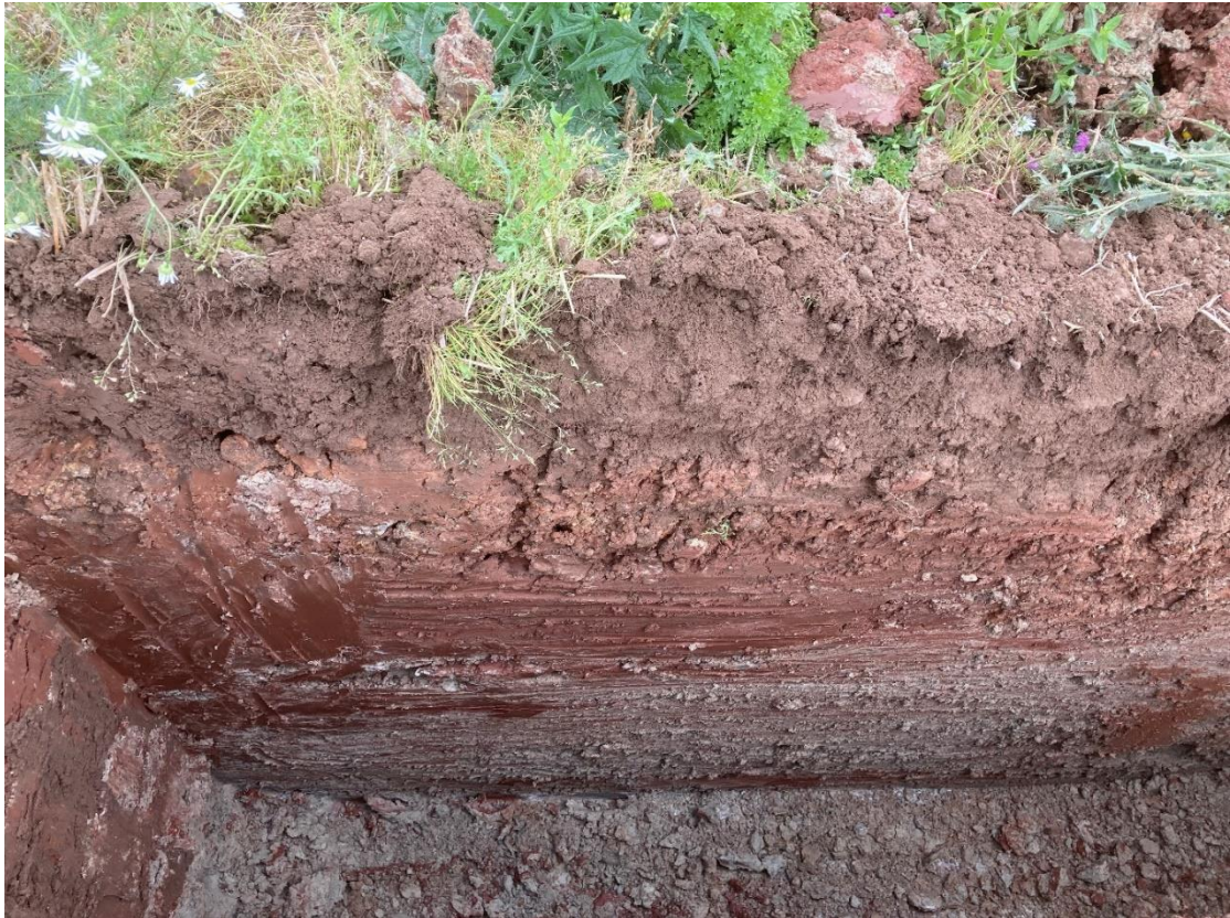
TP06 Trial Pit
