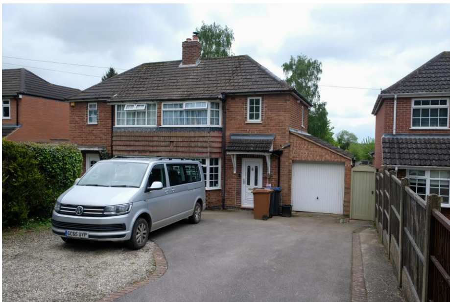
Figure 8 - View of Front of 53 Hollycroft Cres. Showing Garage to be Demolished
