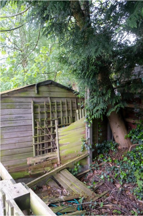
Figure 3 - Sycamore to be removed - Photo 1
