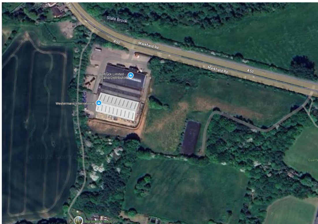
Figure 1: Aerial Image of Site
