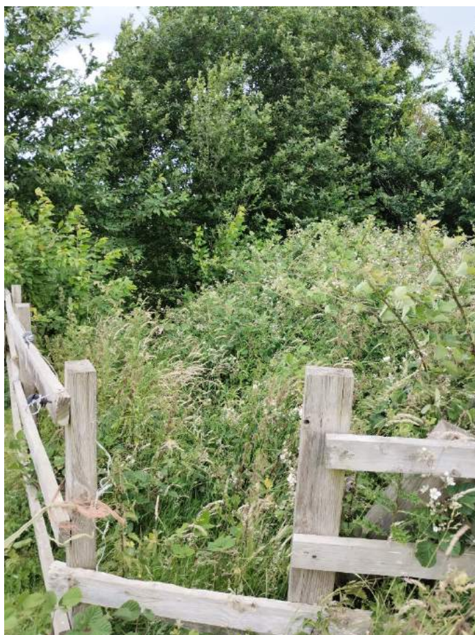
Plate 6: View of the public footpath, looking north; steps with wooden retention beams hidden in the vegetation
