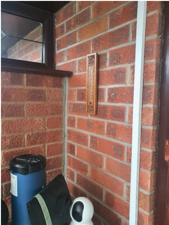
General view of right junction of conservatory to main bungalow – Gap has been repointed
