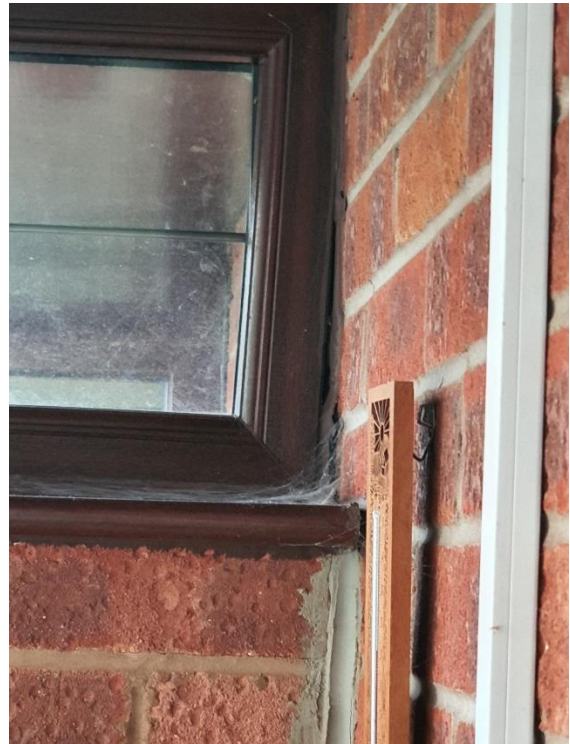
Close view of pulling of the double-glazed frame
