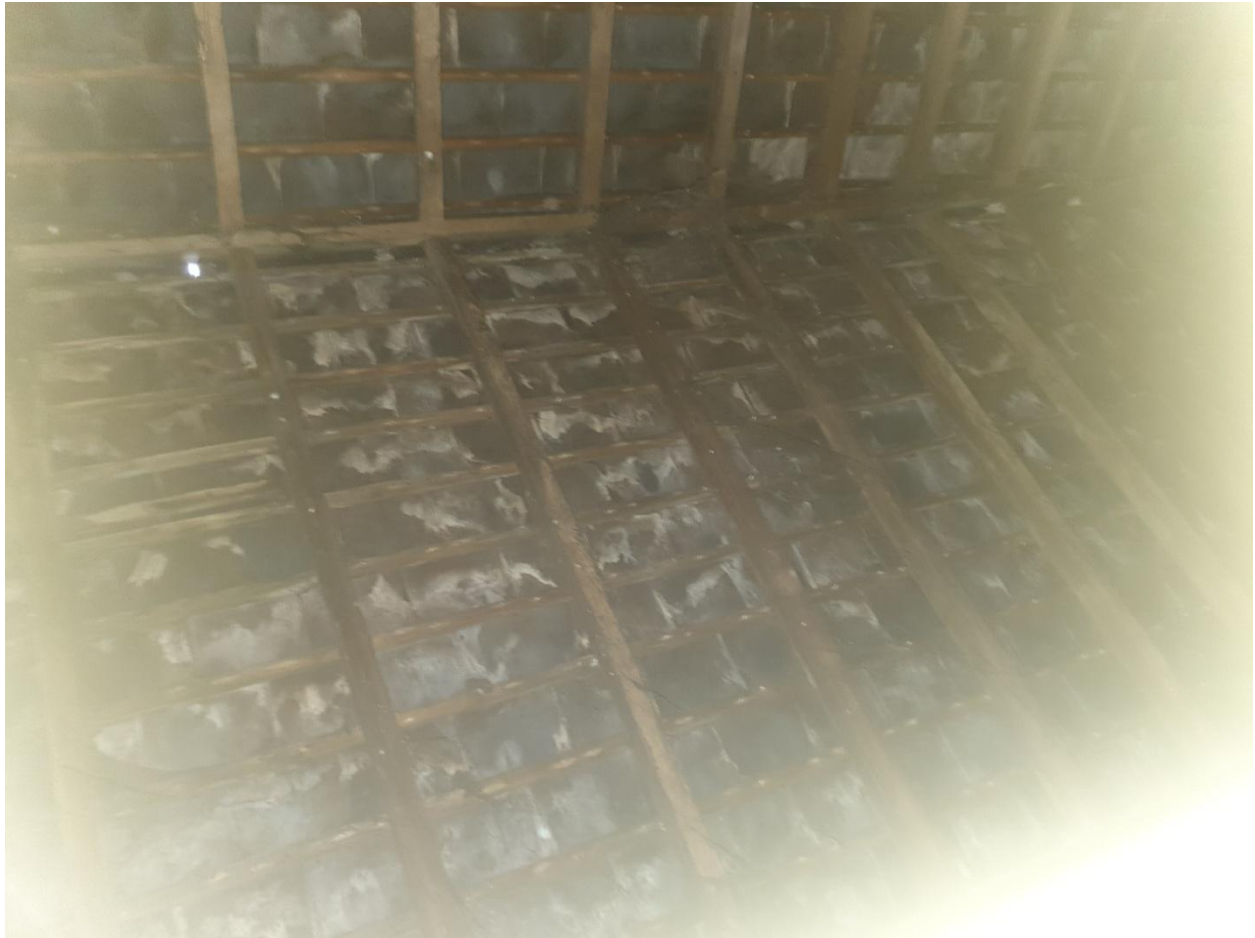
Main roof space: unlined slate
