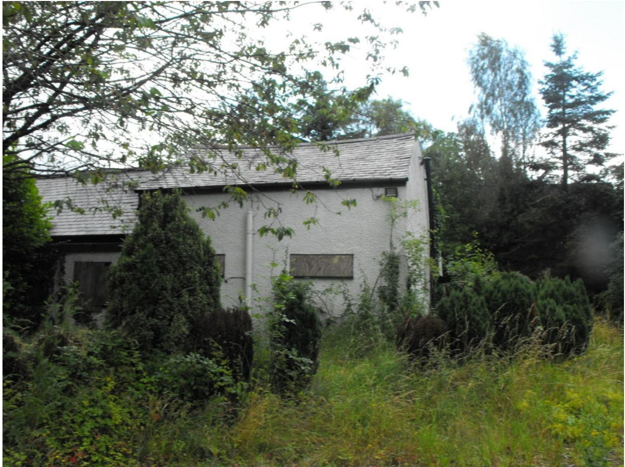
Single storey structure to north
