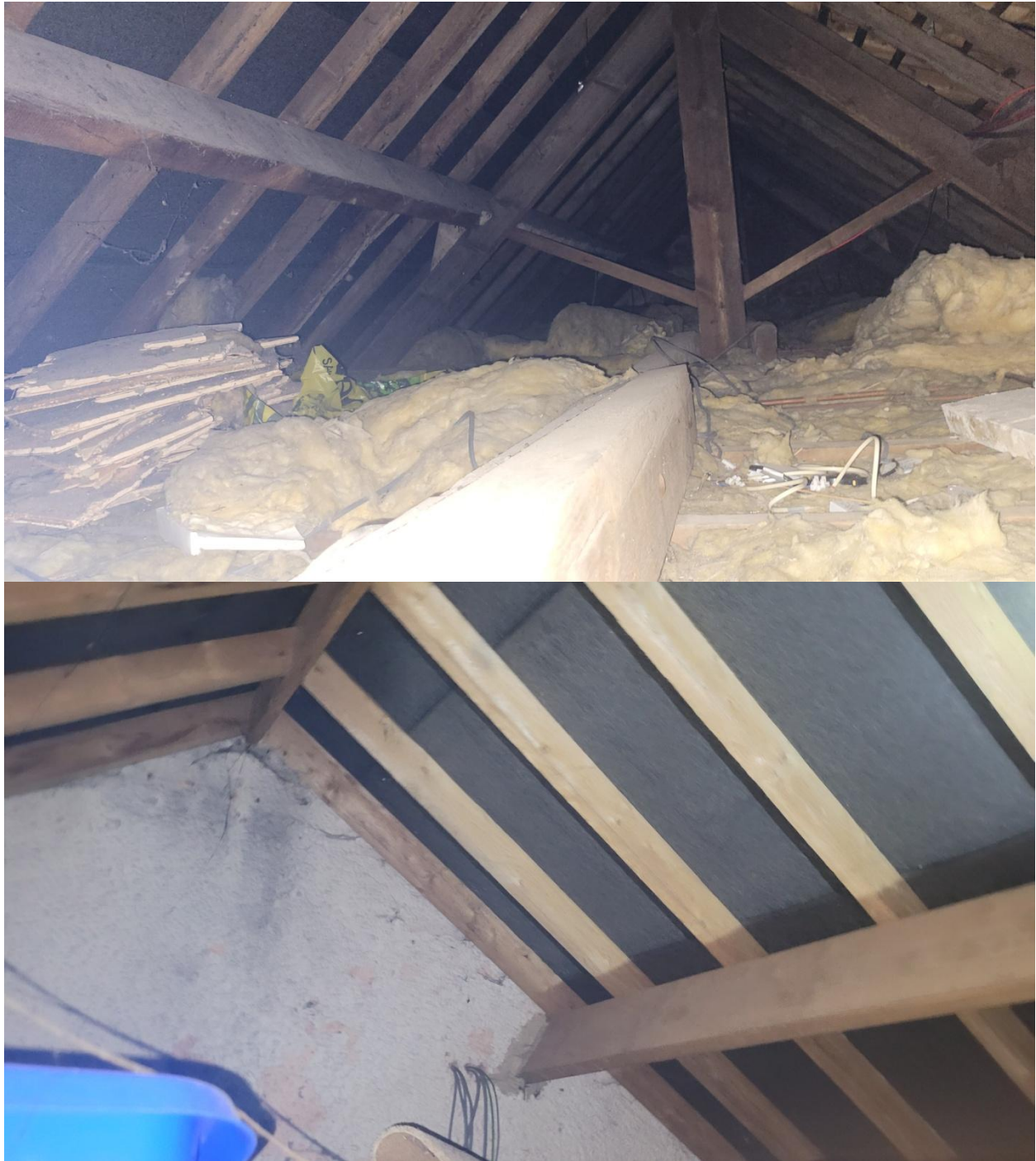
Main loft space of dining area, lining bitumen felt
