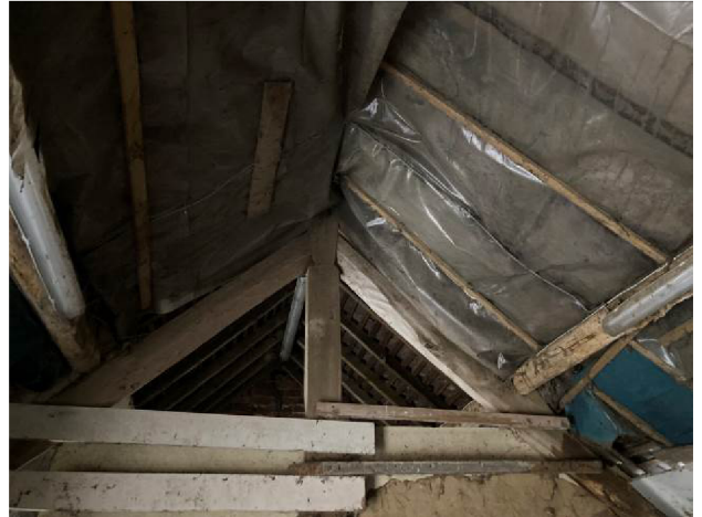
Open underside of roof B2
