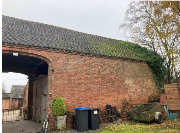
North west side B3
