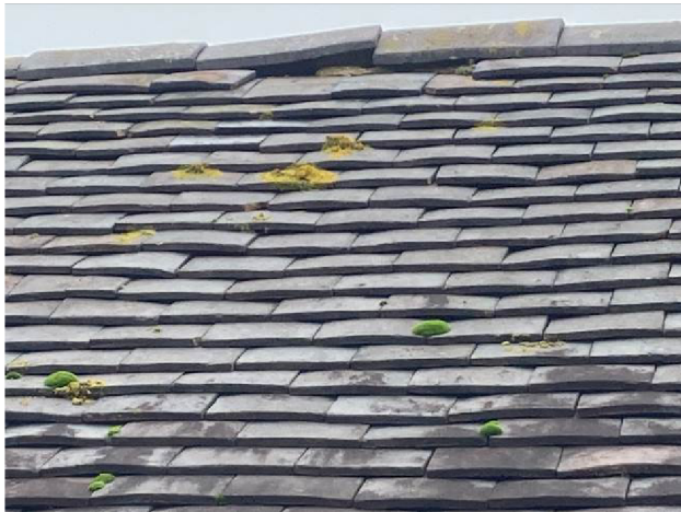
Close up of tiled roof B2
