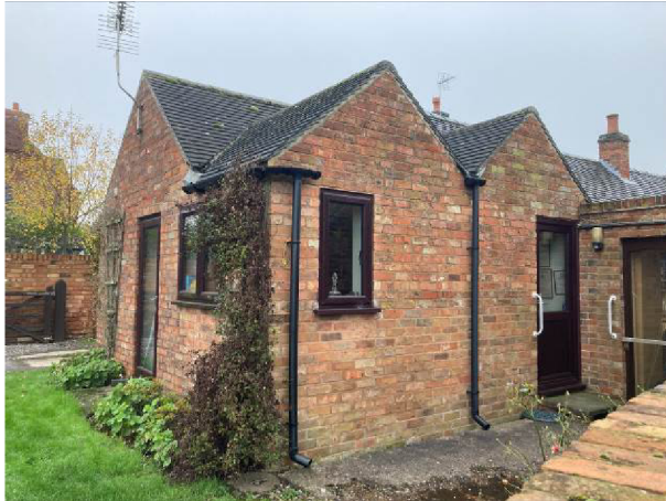
Front (north and west side)
