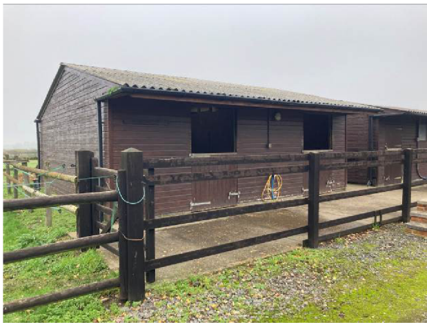
Exterior south face B6
