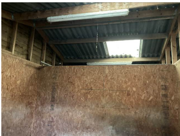
Interior of B6
