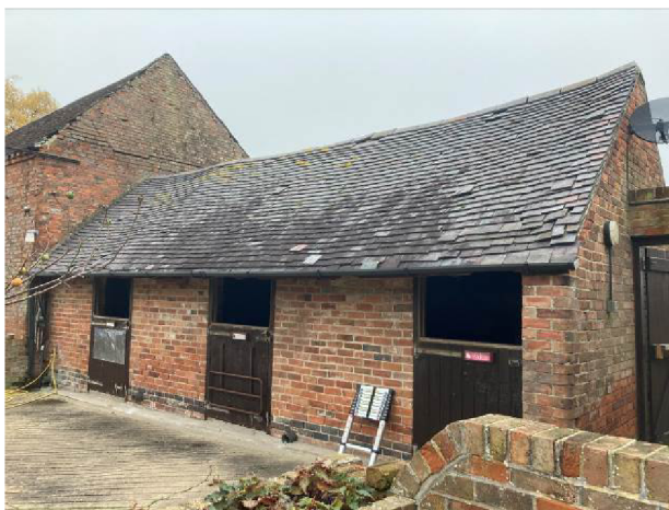
Front (south face) of B2
