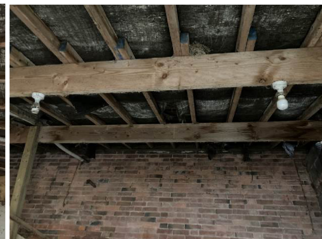
Interior of B4 lean to extension
