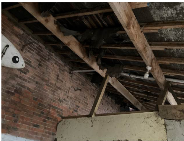
Interior of B4 lean to extension
