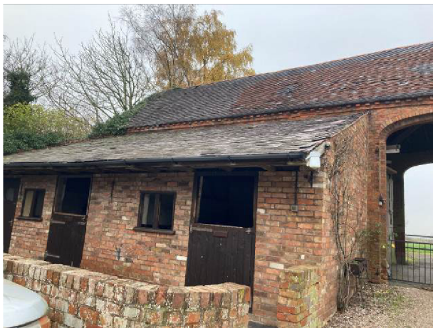
South west side B3 and B4
