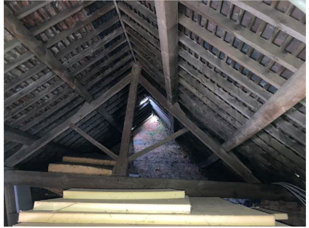
Roof space interior west side
