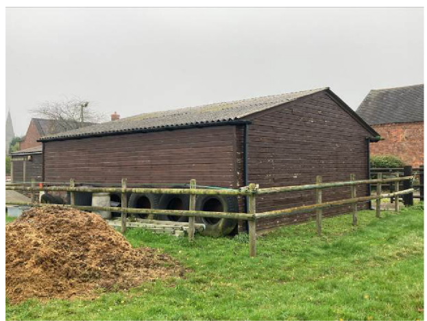
Exterior north face B6
