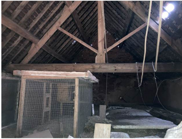
Roof space interior east side
