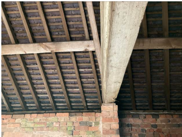
Underside of roof east side
