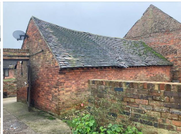
Rear (north face) of B2
