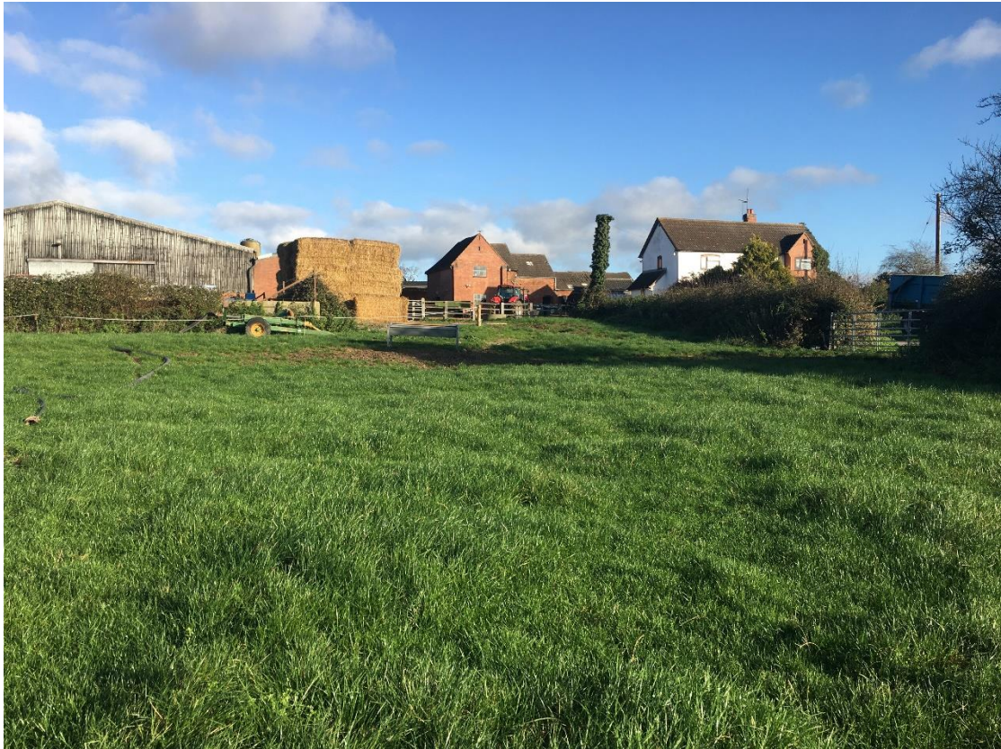
Plate 12: Middlefield Farm from the public footpath running to the west of the farmstead.
