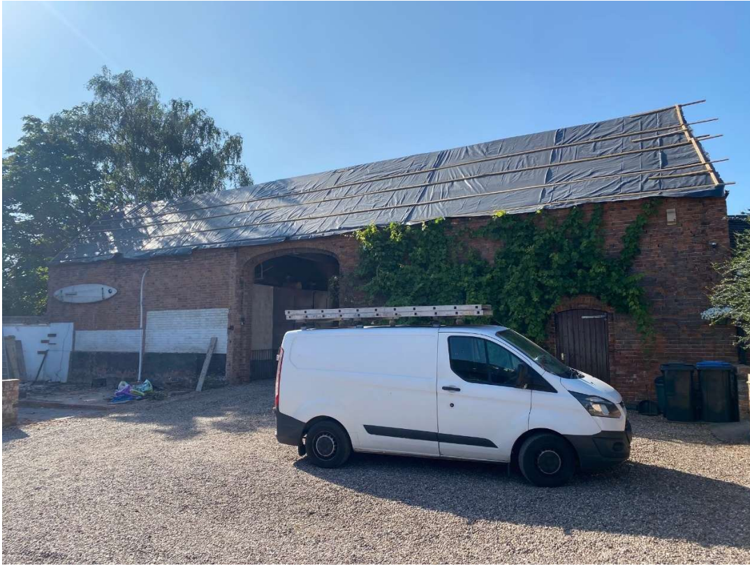
Roof tiles removed from Building B3 (Barn Conversion) and demolition of building B4 commencing the conversion of Building B3 and associated replacement roof.
