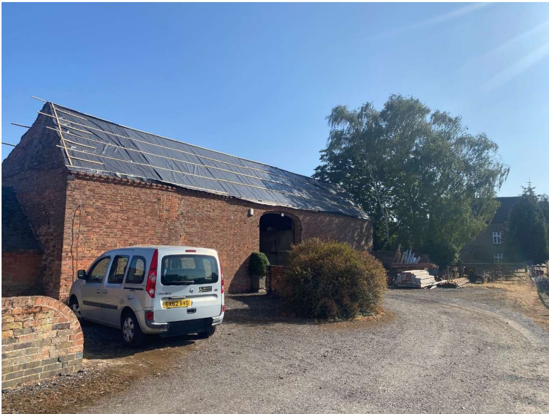
Roof tiles removed from Building B3 (Barn Conversion) and demolition of building B4 commencing the conversion of Building B3 and associated replacement roof.
