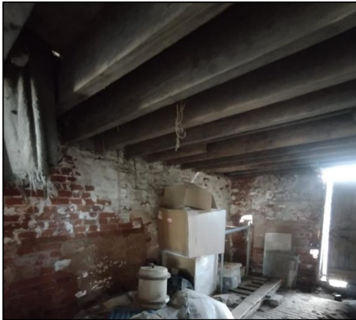
Photograph 5: Representative image of the ceiling structure of the barns lower level.
