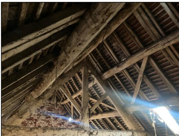
Photograph 7: Roof structure of the eastern and midsection of the upper floor of the barn.
