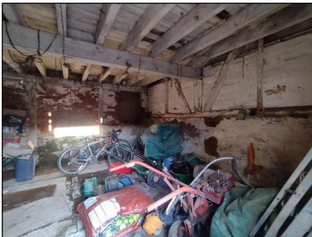
Photograph 3: Room of the lower level used for storage
