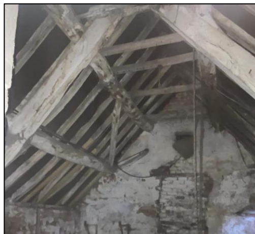
Photograph 8: Roof structure of the western section of the upper floor of the barn, with bitumen felt present.
