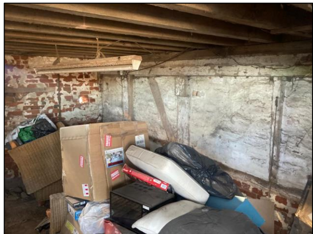
Photograph 4: Room of the lower level used for storage
