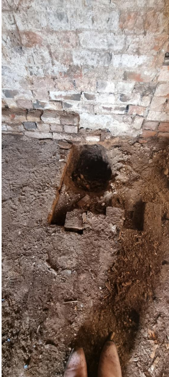
FOUNDATION TO REAR WALL
