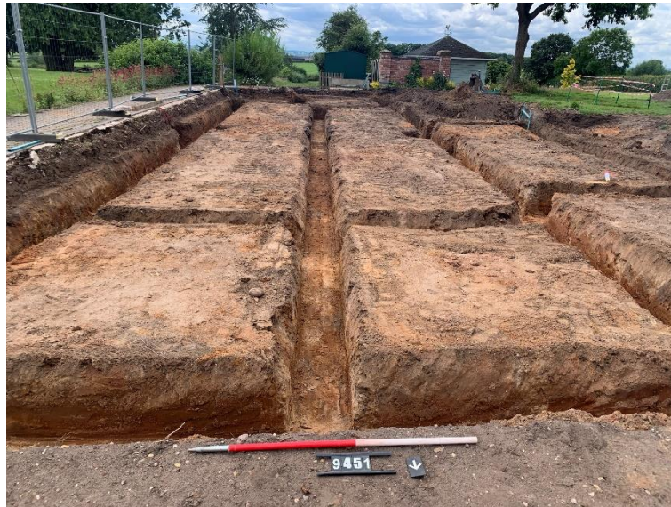
Plate 1: Overview of the excavated footings, looking south, 1m scale
