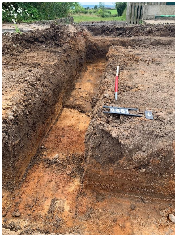
Plate 4: Shot of southern end of building footings, showing levelling layer (1004), looking south, 1m scale
