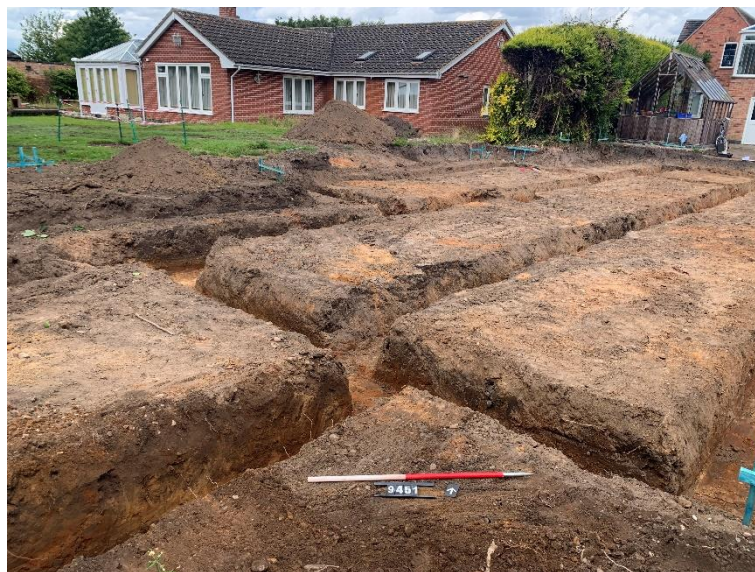
Plate 2: Overview of the excavated footings, looking north, 1m scale
