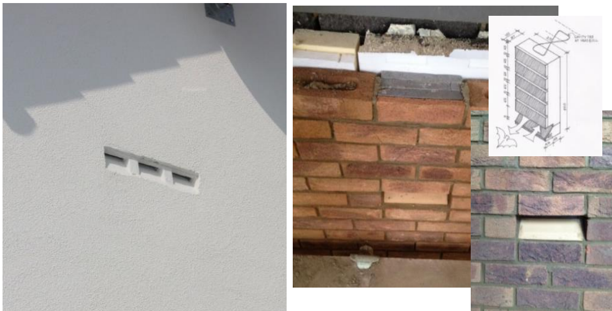
Figure 3: Examples of bat tubes fitted within the brickwork of an exterior wall.
