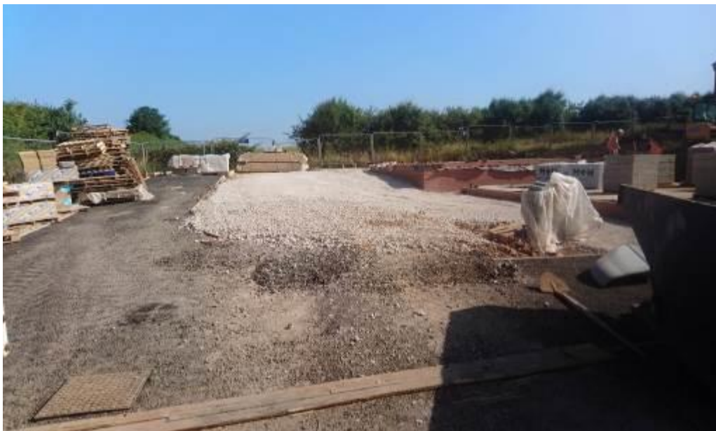
Placement of stone to the front of plots to create clean forklift access
