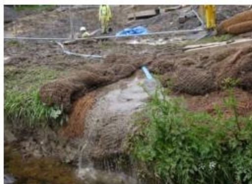
Deployed to treat muddy excavation water
