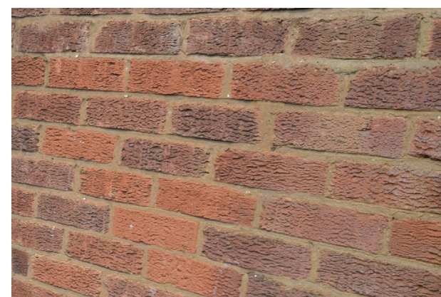
04 – Existing facing bricks.
