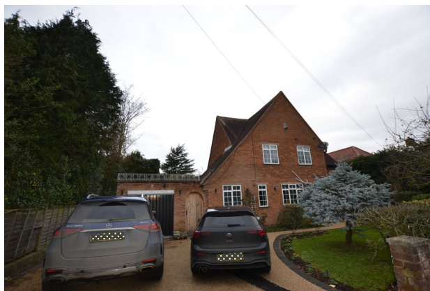
01 – Front elevation of existing dwelling.
