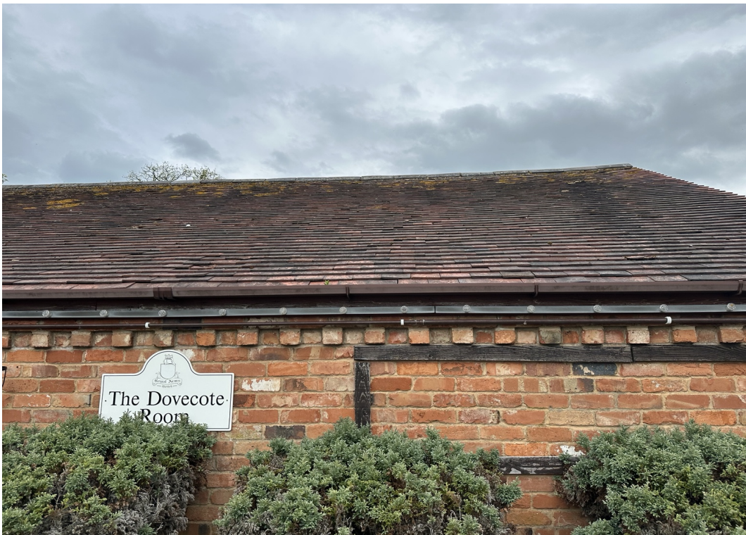
Existing reclaimed roof tile appearance
