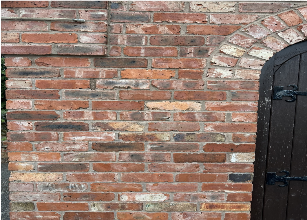
Existing brickwork and detailing
