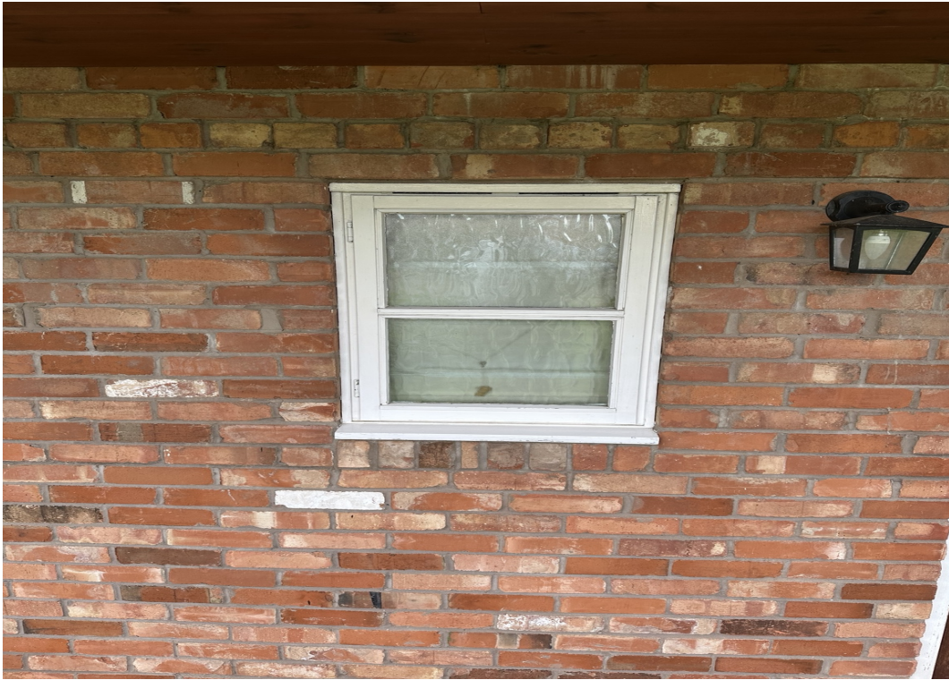
Existing white painted timber window detail
