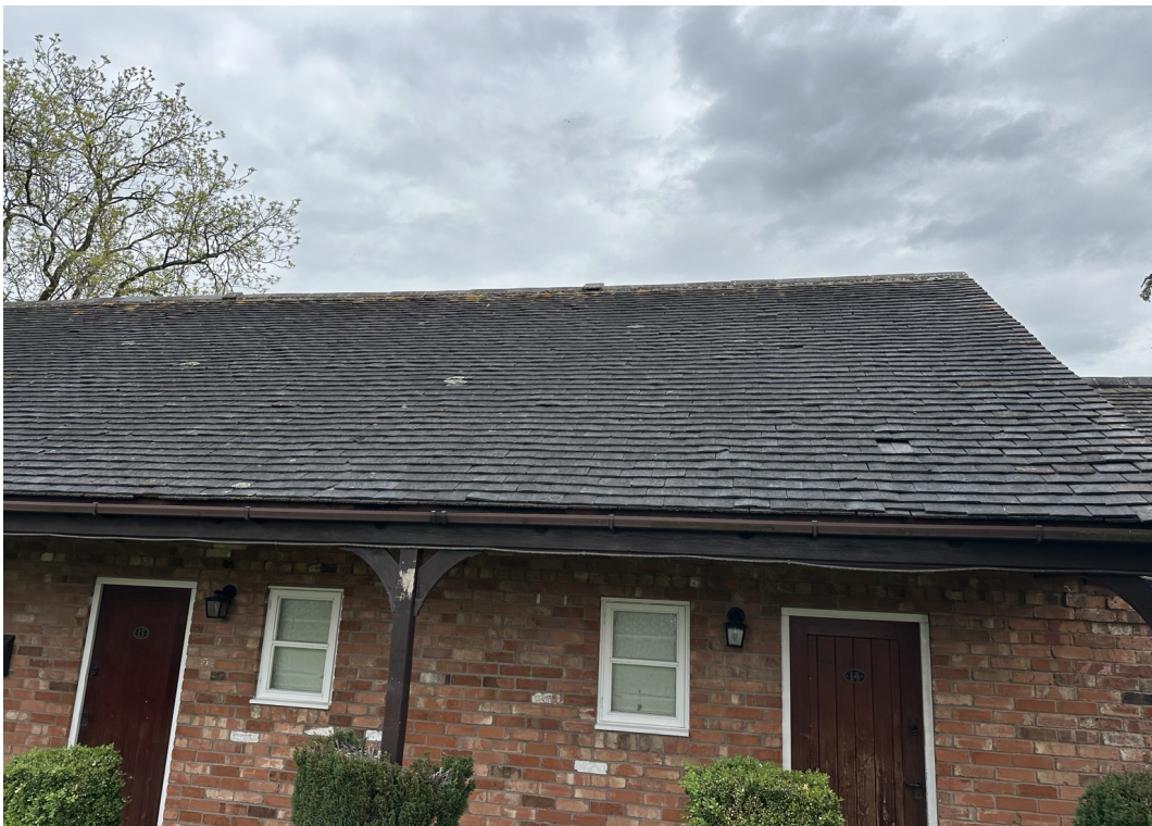
Existing roof and external appearance
