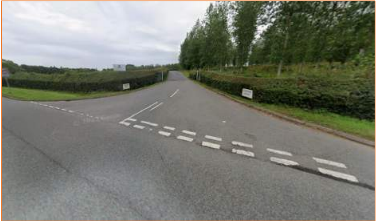
Figure 10: Existing Horsepool Grange access road, with the Eliotts Lane junction in the foreground
