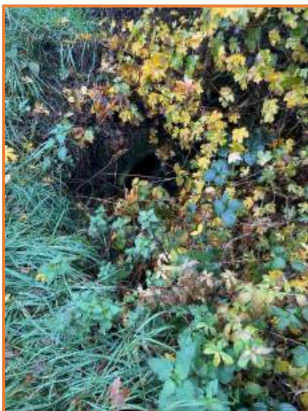
Figure 11: Culvert under existing access to Horsepool Grange industrial estate.
