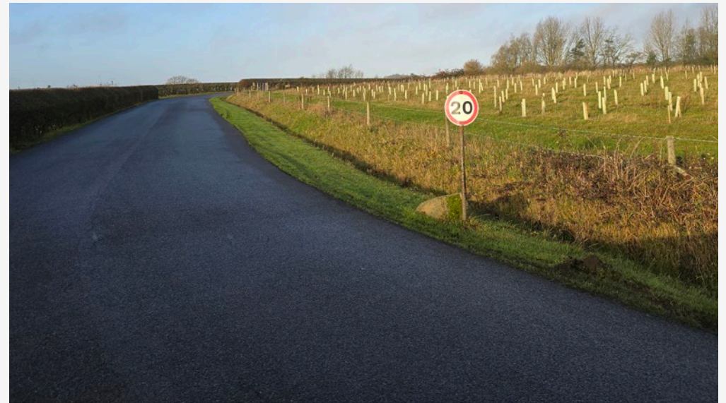
View toward west of the site from access road
