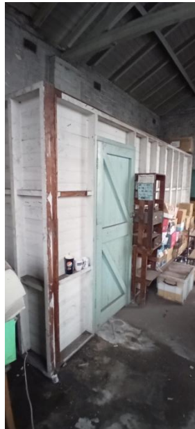
Internal View of roof structure with modern electrical fittings
