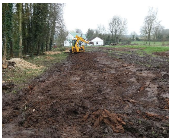
Figure 15: General view north after backfilling
