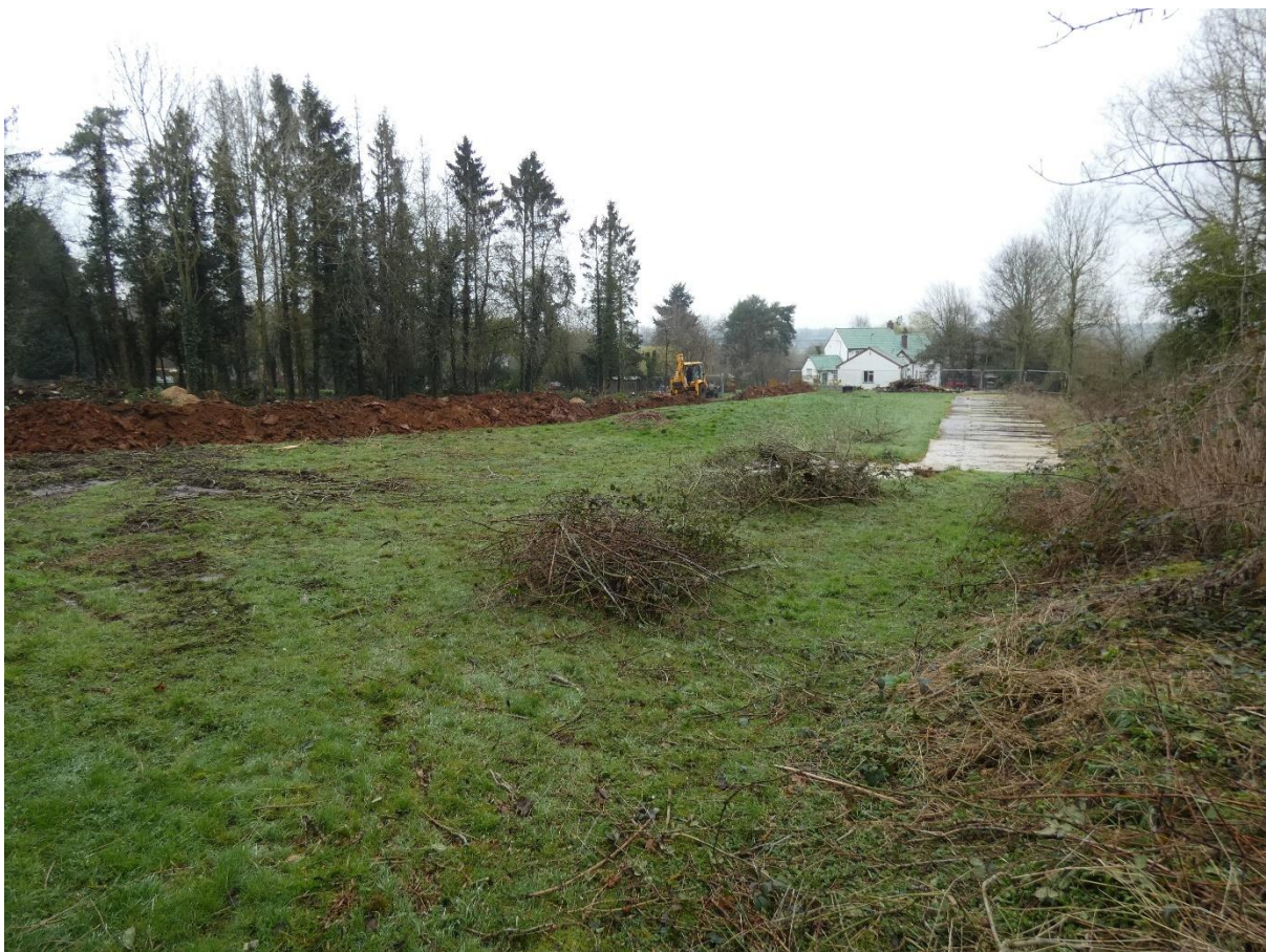
Figure 4: The site with trenching underway, looking north.
