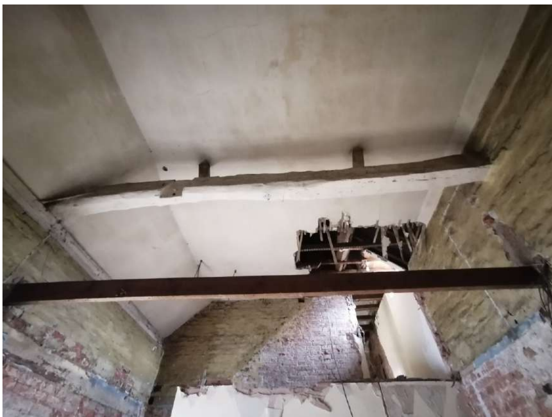
Plate 17; east-wing of re-used timber recorded in the former Moore's Arms showing possible re-used cruck.
