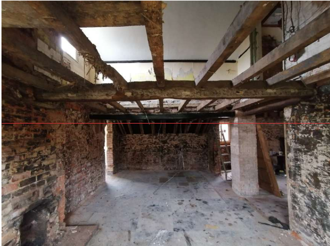
Plate 18; west-wing of re-used timber recorded in the former Moore's Arms showing re-used C17 wall-frame beam with mortices for square-panel framing.
