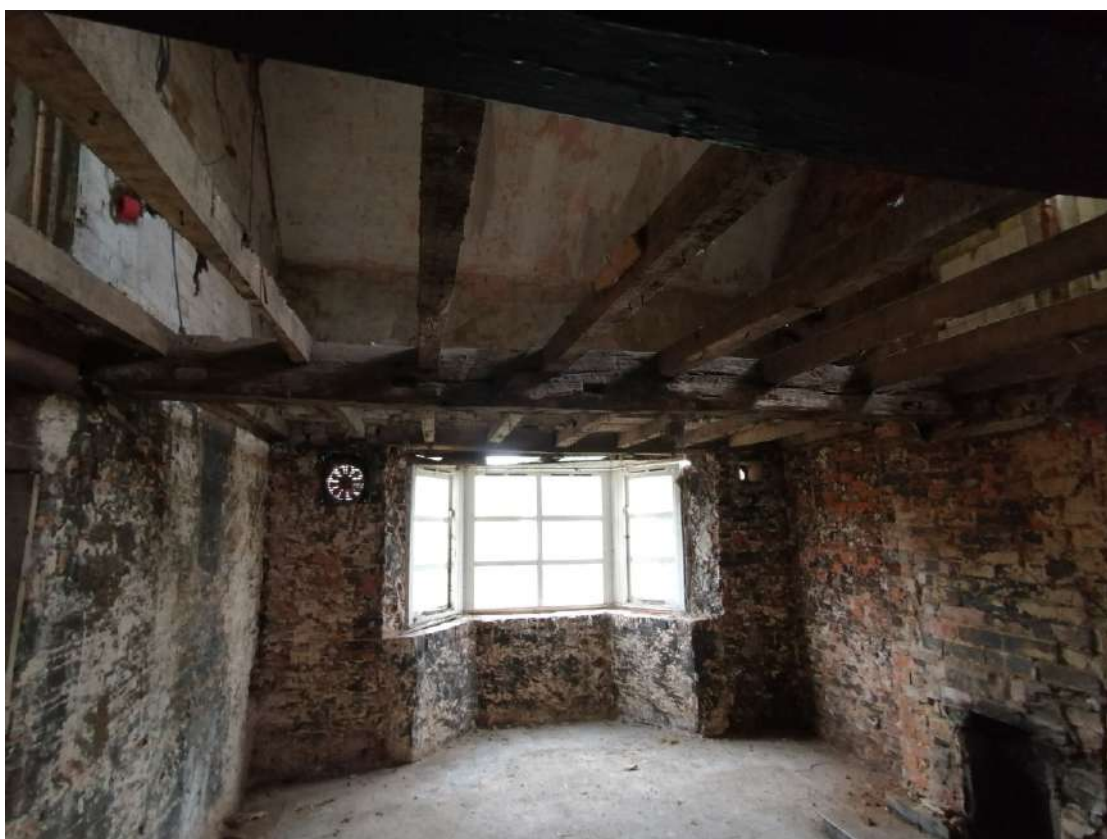
Plate 17; east-wing of re-used timber recorded in the former Moore's Arms showing possible re-used cruck.
