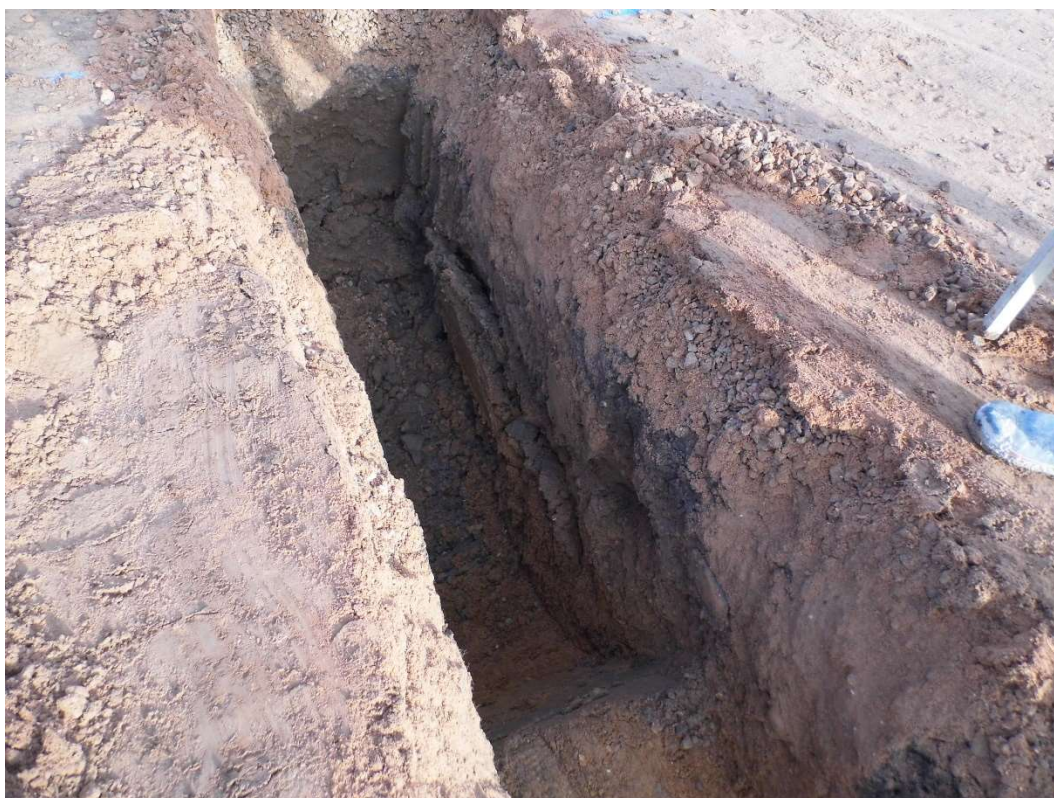
Figure 15: North-eastern ditch [28] along north-west foundation trench partially excavated looking north-west
