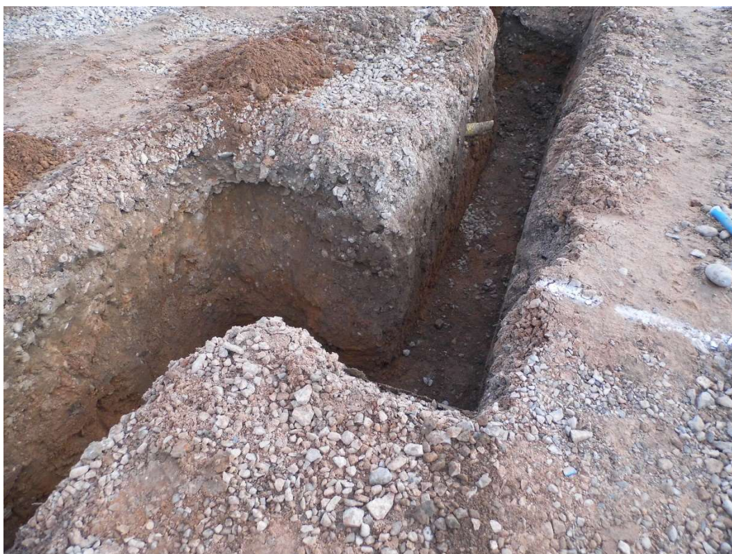
Figure 22: Gully [30] in Plot 2 middle foundation trench showing section looking north
