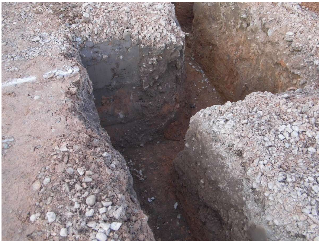
Figure 23: Gully [30] in Plot 2 middle foundation trench showing section looking south-west
