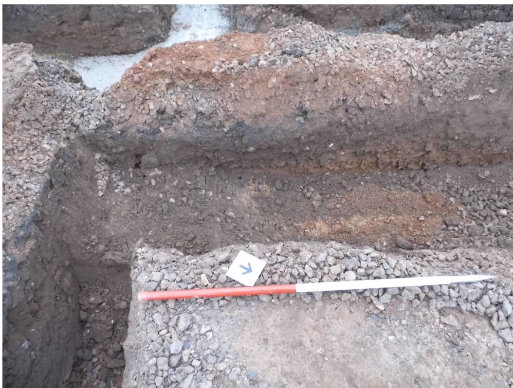
Figure 26: Gully [30] in Plot 3 north-west foundation trench looking south-west
