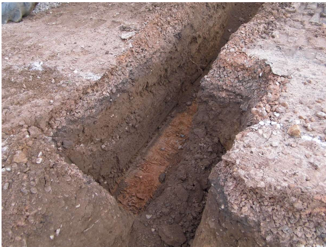
Figure 28: Gully [30] in Plot 3 middle north-west to south-east foundation trench looking north
