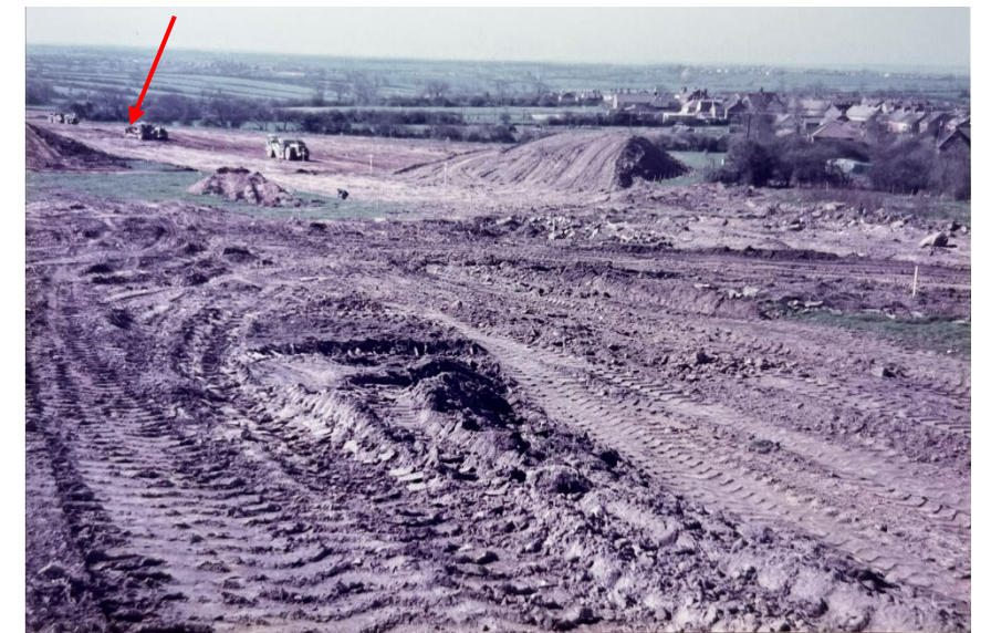
Plate 4: Late 20 th century photo of works at Cliffe Hill Quarry depicting Site to the left.
