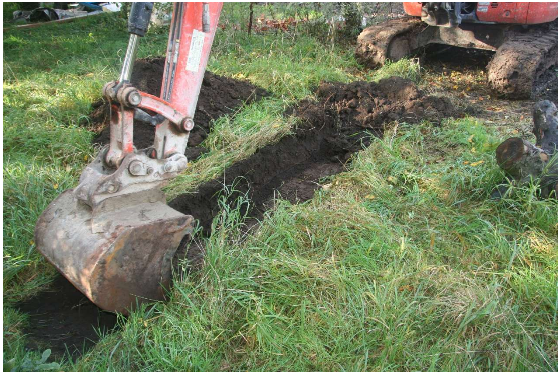
Plate 1: Working view of the monitored groundworks, looking North.
