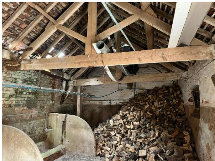
Plate 7: Building B1 internal
