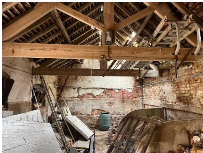
Plate 8: Building B1 internal
