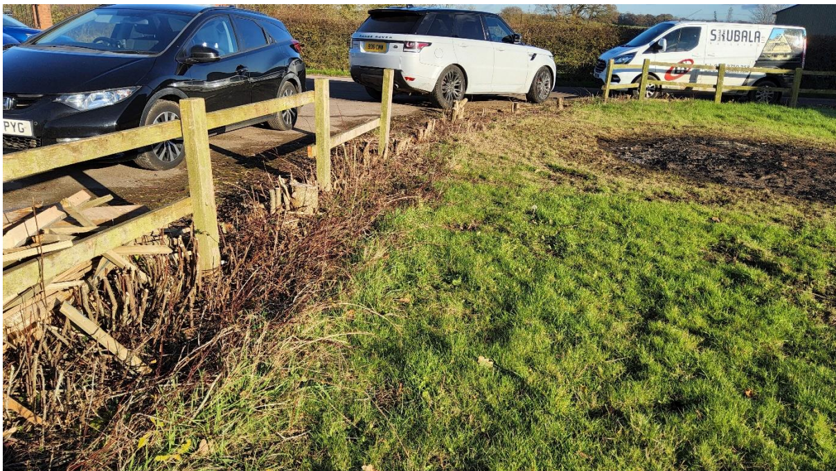
Photo 7. Recently removed remainder of H1, looking east
