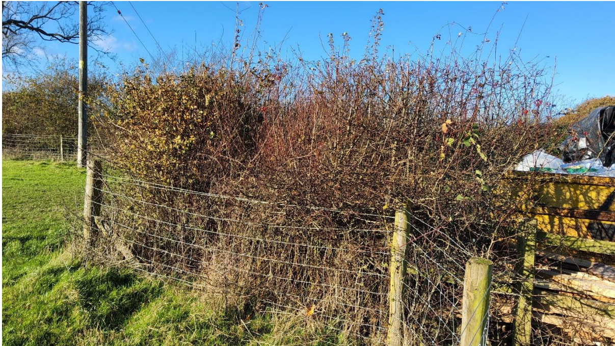
Photo 6. Retained section of H1 in the northwest
