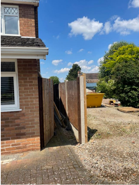
Figure 1- Fence separating no.67
