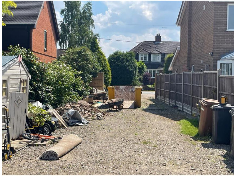
Figure 4 - View from access looking towards Main Street
