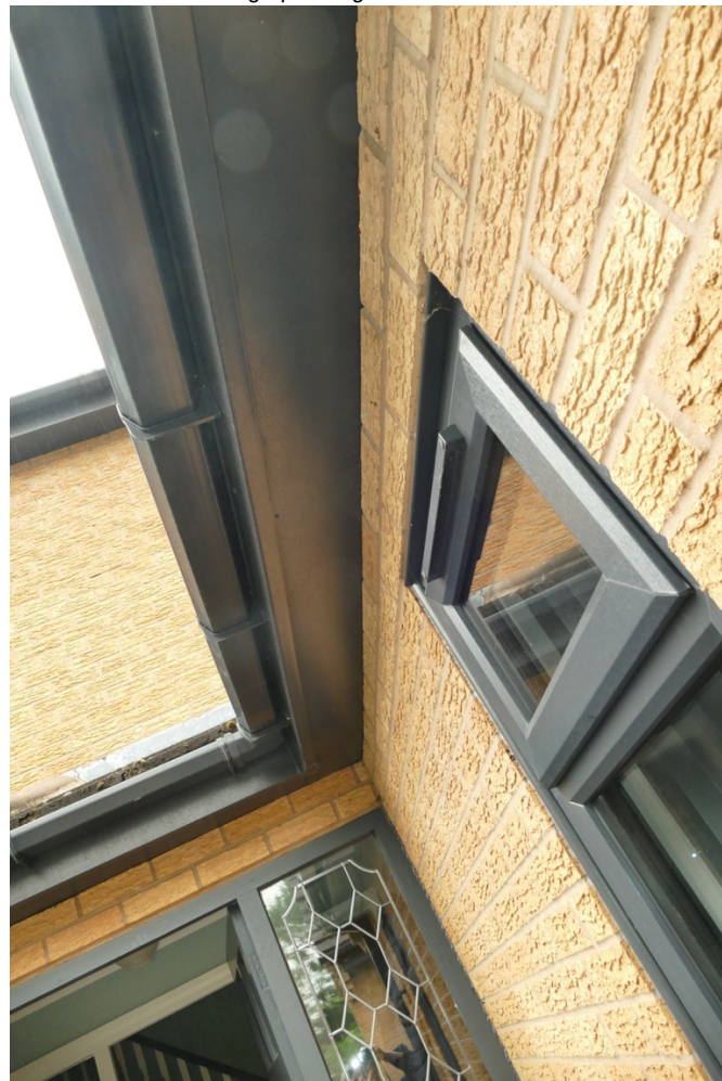
Photograph 3 – general soffit detail
