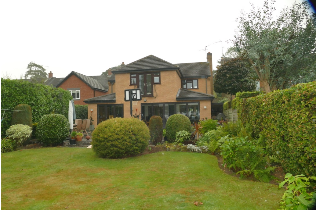
Photograph 2 – dwelling, rear, northwest facing aspect.
