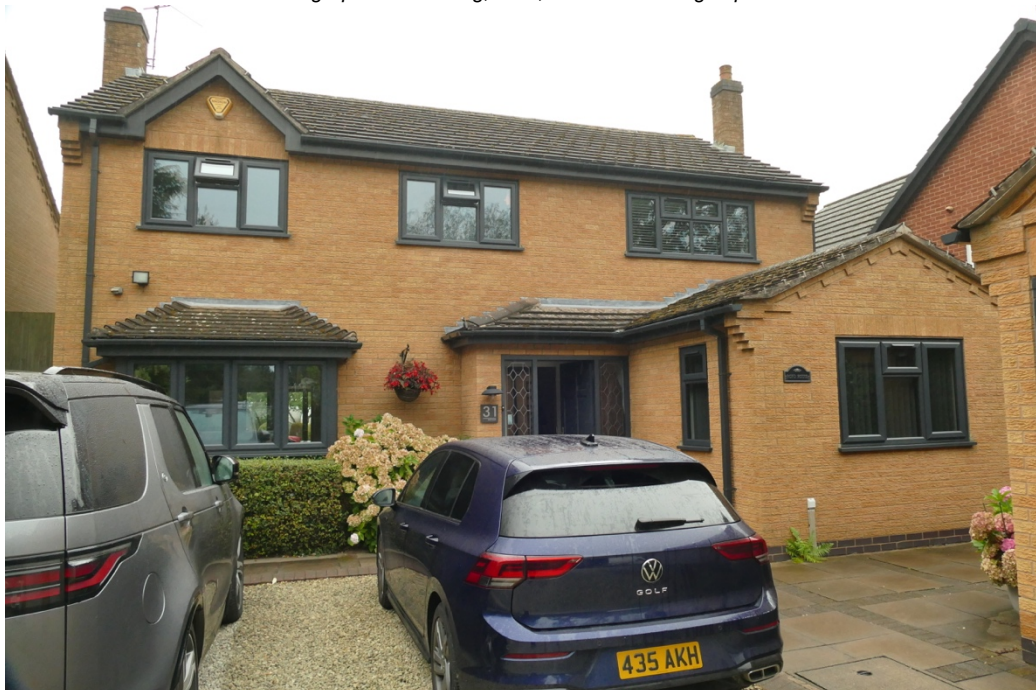
Photograph 1 – dwelling, front, southeast facing aspect.
