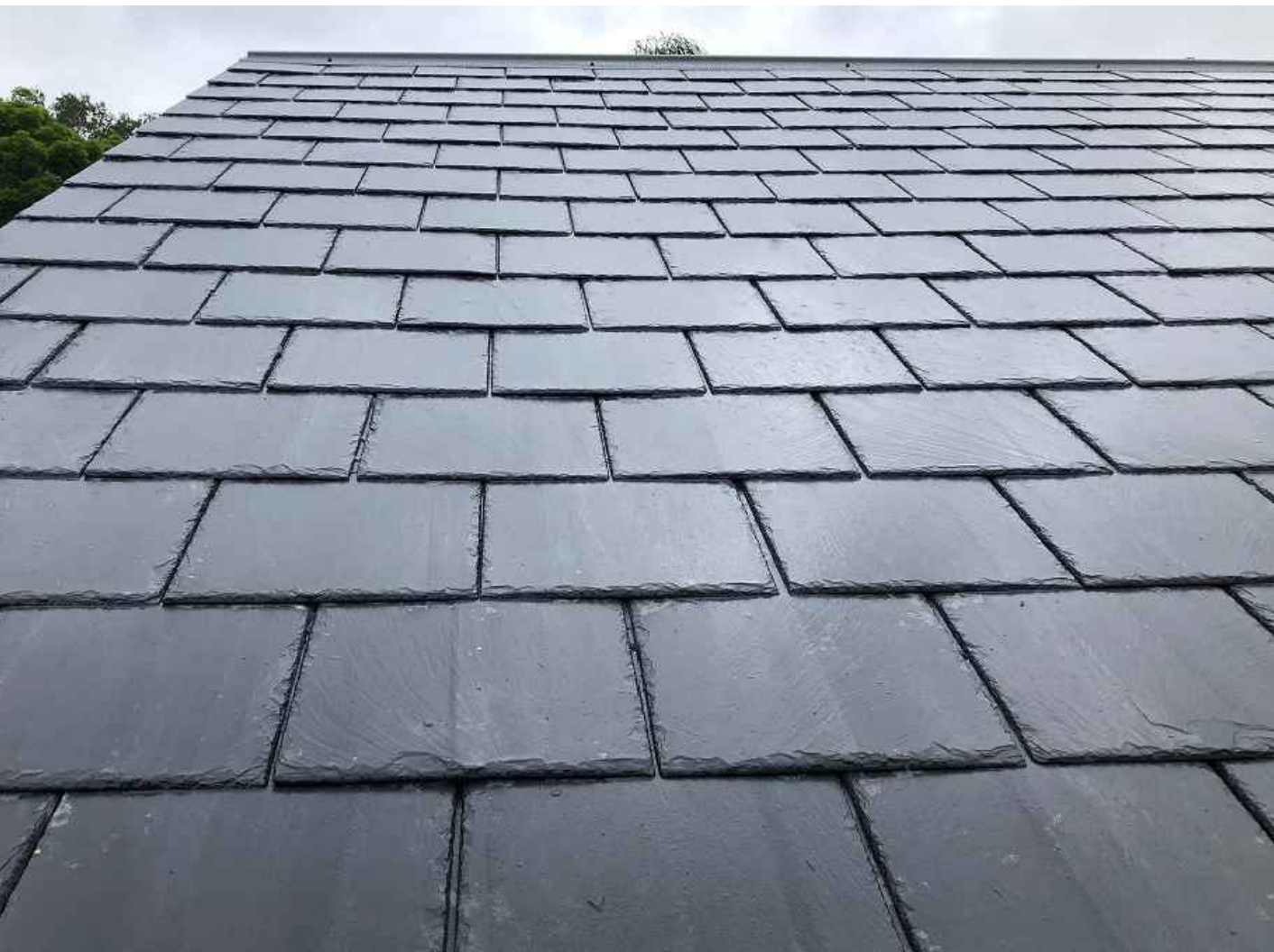
Example Roof Covering
