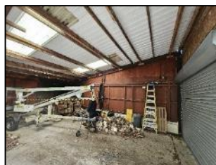
North aspect of the building.
