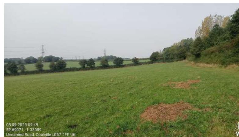
Figure 2: Northeast of site (looking west) - The new main bund will separate Unit 1 and 2 from the grassland and balancing ponds to the east. The land slopes to the south so material will be cut from the upper slopes to the north (right of photo) and filled to the south (left of photo).
