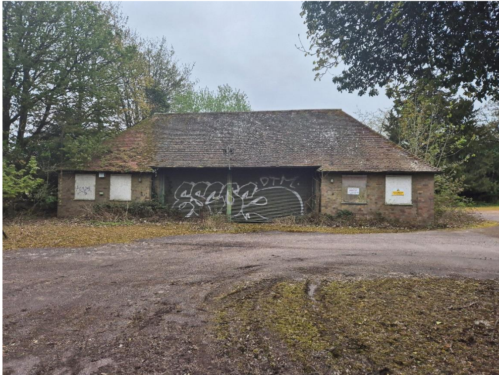
External View of Garage Unit
