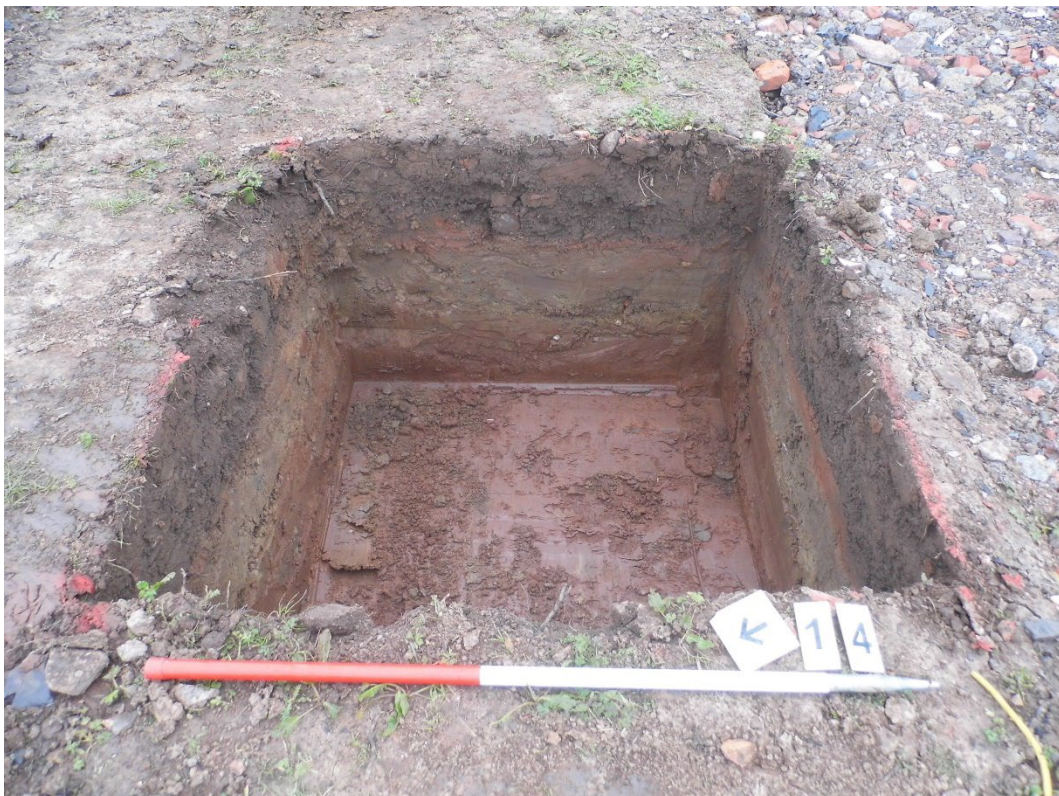
Figure 15: Pad pit 14 looking south-east
