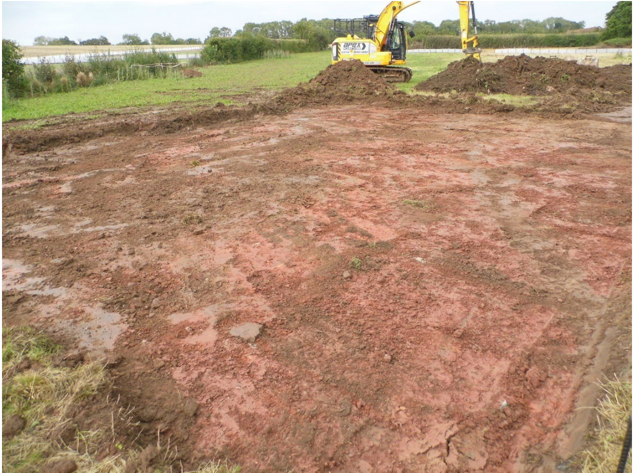
Figure 6: Compound strip looking north
