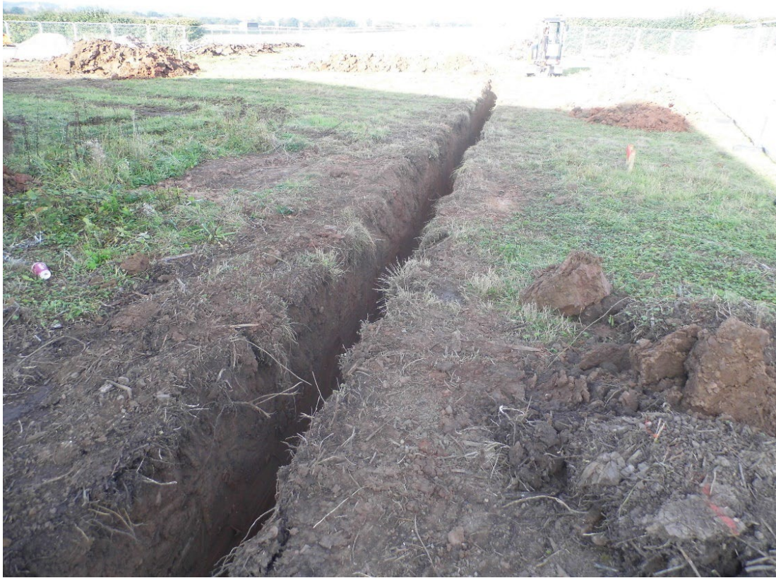
Figure 7: Excavated drain trench
