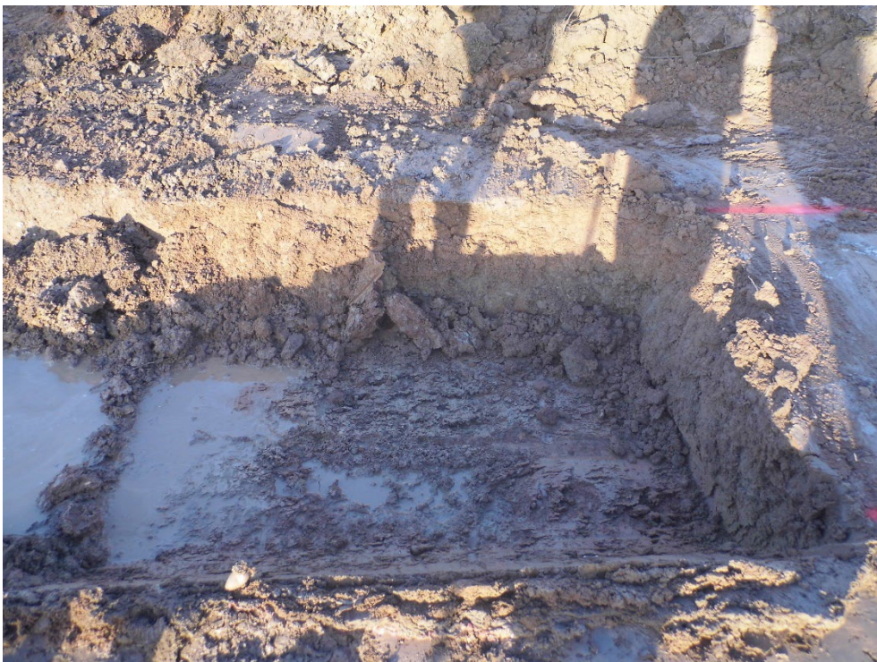
Figure 11: Eastern foundation trench looking north-east
