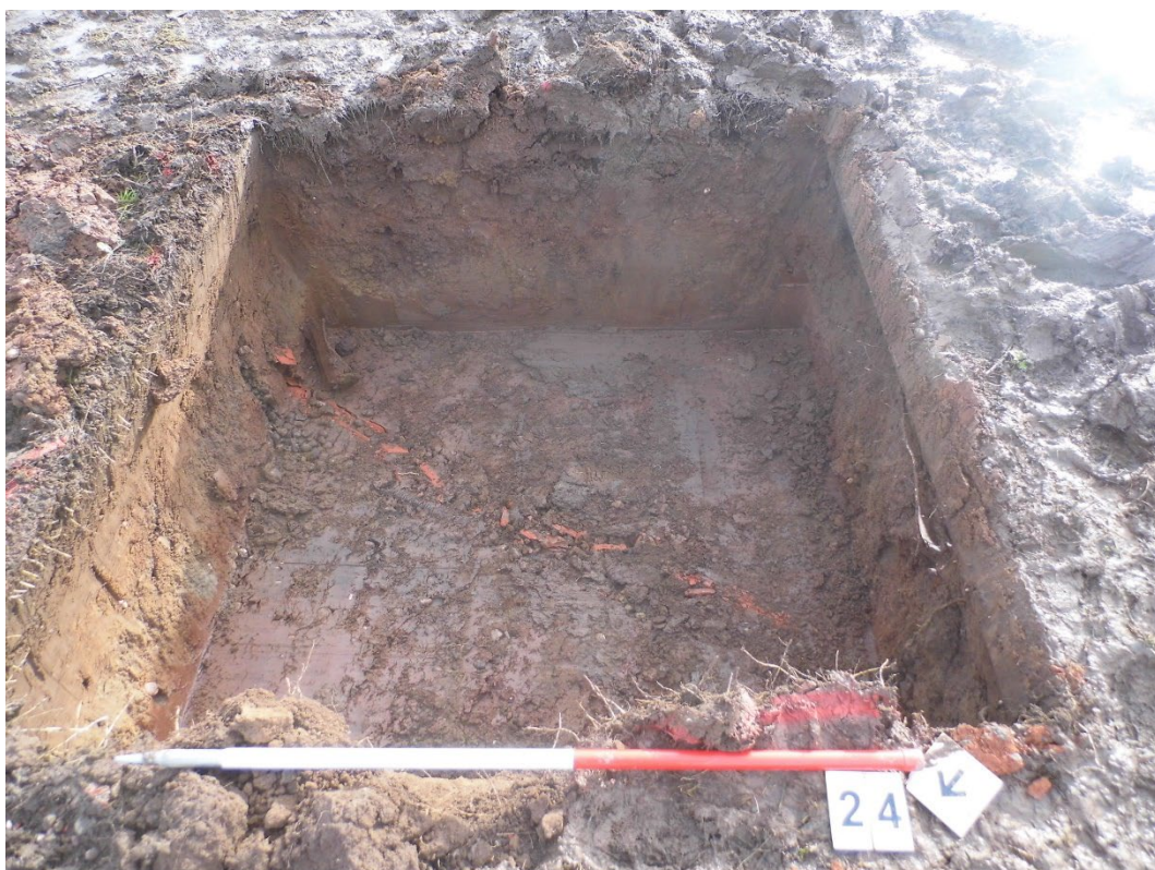
Figure 20: Pad pit 24 looking south-east
