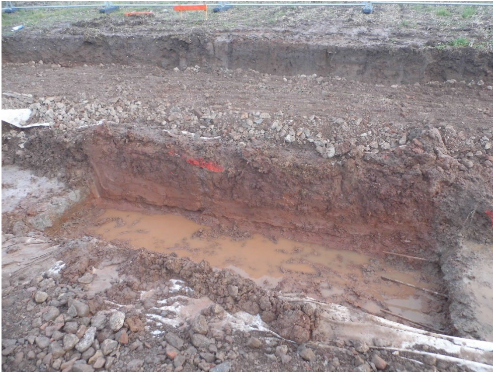
Figure 10: North-west foundation trench looking north
