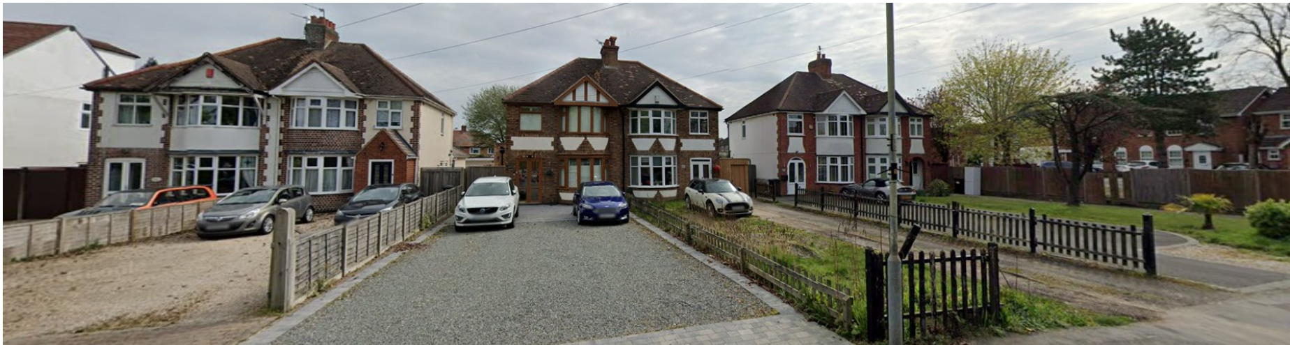
Photo 2—Easterly View along Rugby Road to the north of The Ridgeway. Traditional 1930's era semi detached two storey dwellings with hipped main roof arrangement and gable detailing. Mix of facing brick and render external wall finishes with brick detailing.
