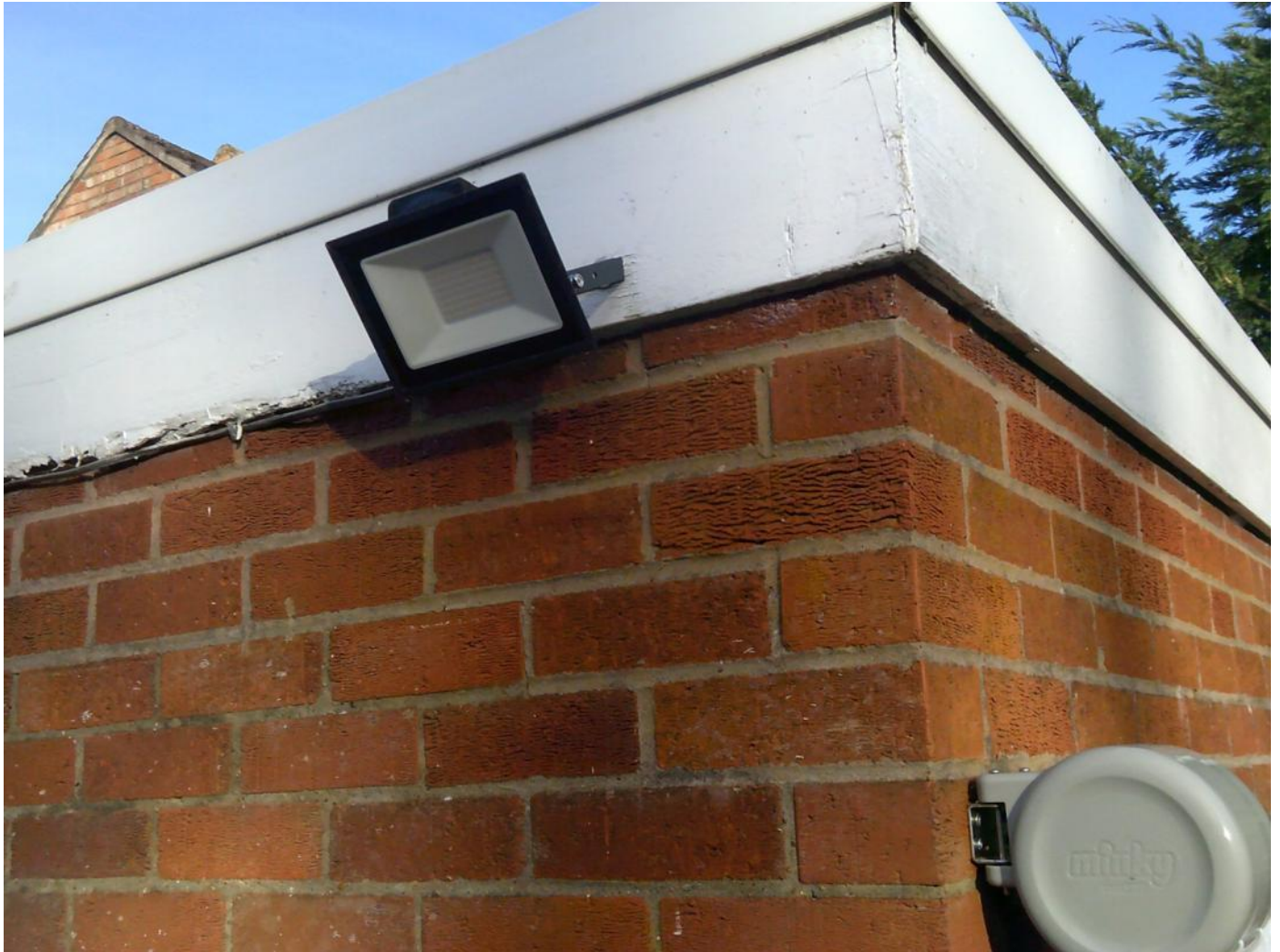
Painted wood soffits on garage
