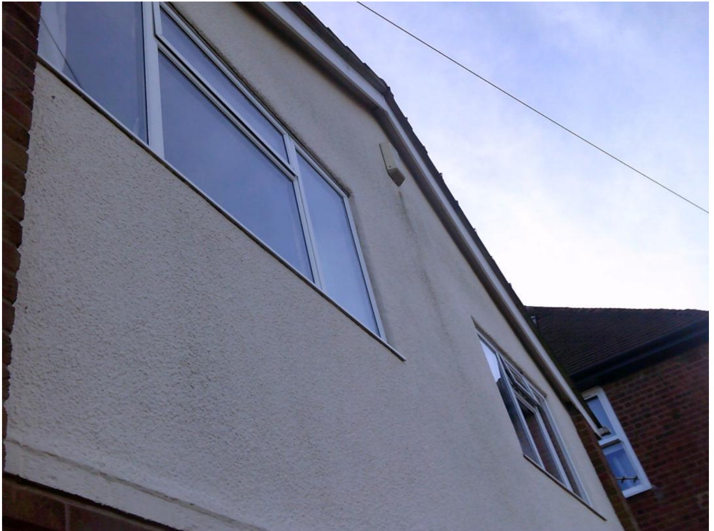
Front elevation intact
