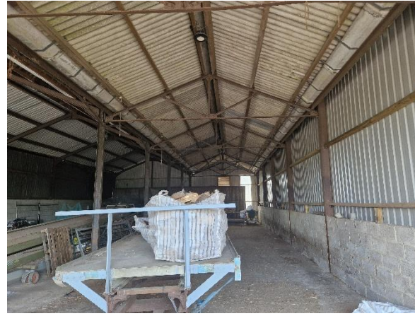
View of internal trusses and columns
