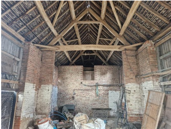
Trusses and internal view in threshing barn
