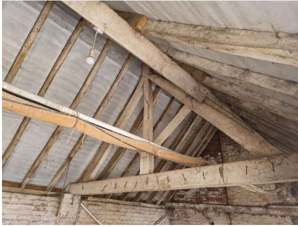
Trusses to single storey Barn
