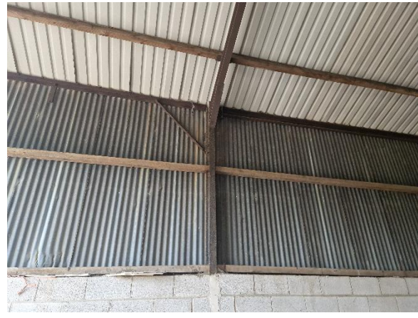
Knee brace at eaves
