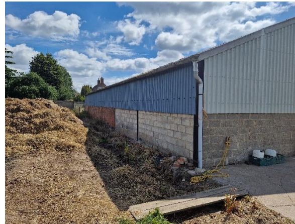
Full side elevation with brick and block
