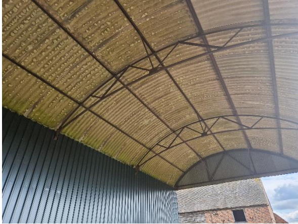
View of roof structure and trusses
