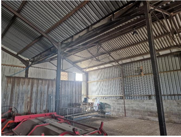
Typical internal view from Barn 3
