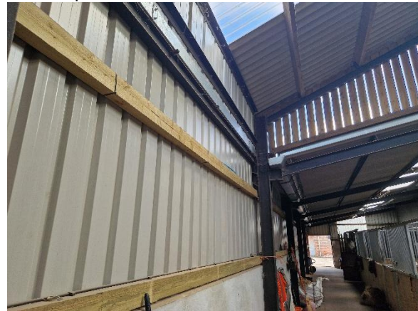
Wall cladding panels and timber rails
