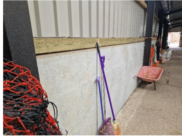
Precast panels at the base of the walls
