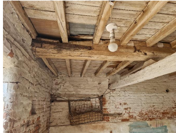
Floor in two storey elements of building
