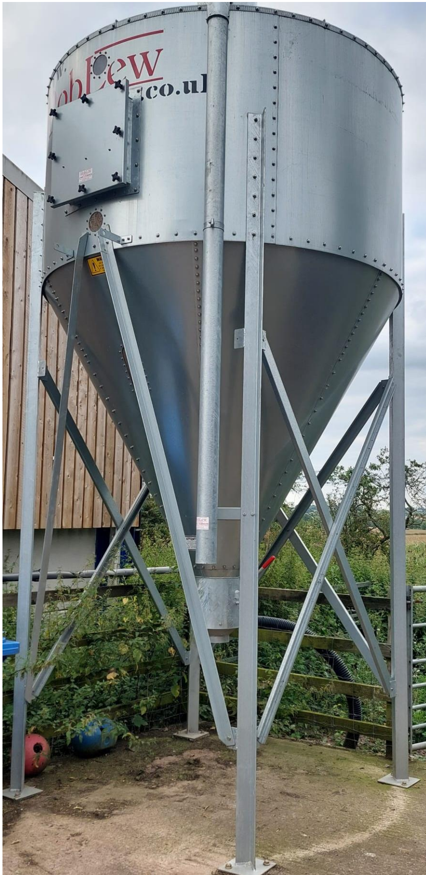
Figure 5 New feed silo adjacent to barns.
