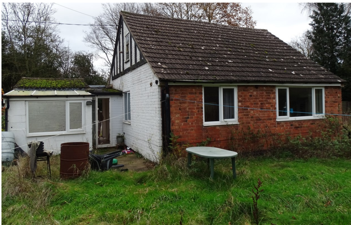
Image 6 – Rear West facing elevation of the property
