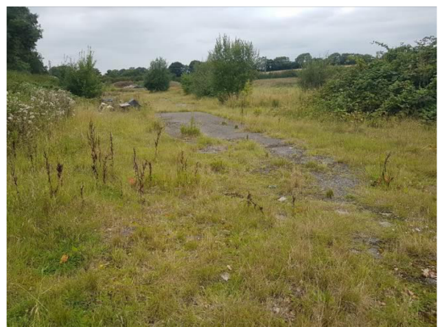
12. Former access road and emerging vegetation
