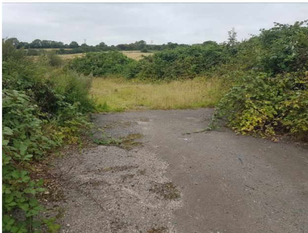
7. Dense scrub and hardstanding on former access road and entrance to the east
