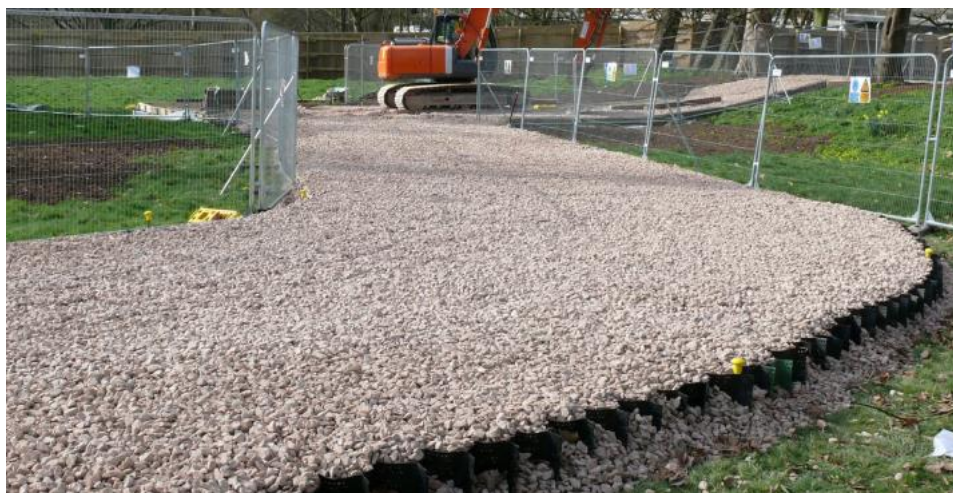
Figure 4 - Example of temporary Cellweb® construction solution
