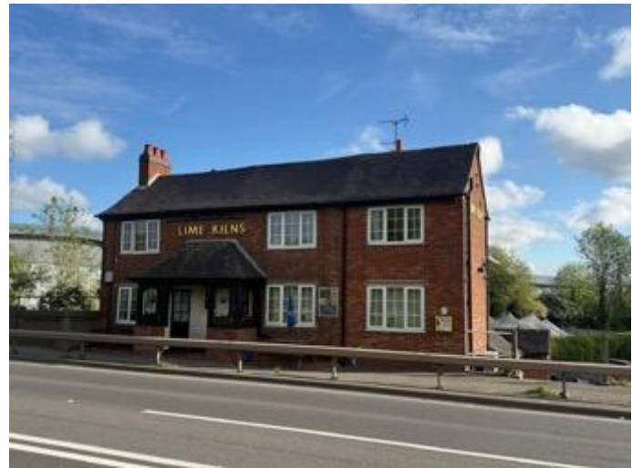
Southern elevation of B1
