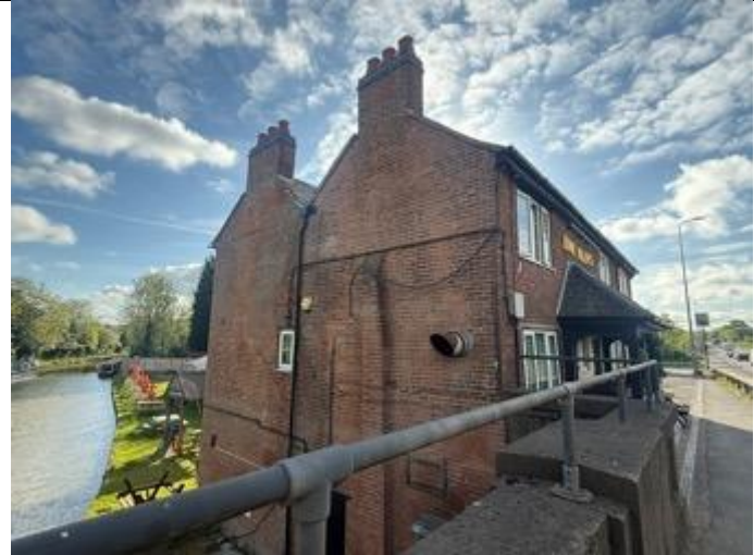
Western elevation of B1
