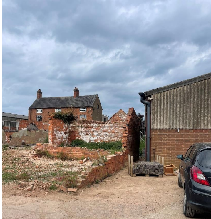
Figure 5 – Photograph of the barn as existing in relation to the Farmhouse
