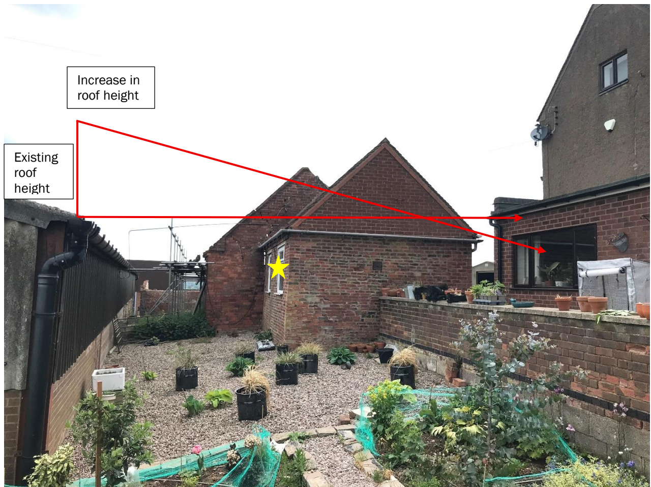
Figure 8 – Photograph showing the relationship between the farmhouse and the barn
