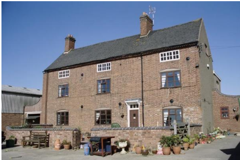
Figure 10: Photograph of Hill Farmhouse
