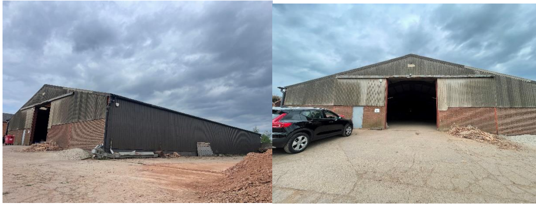
Figure 1 – Photographs of the barn as existing
