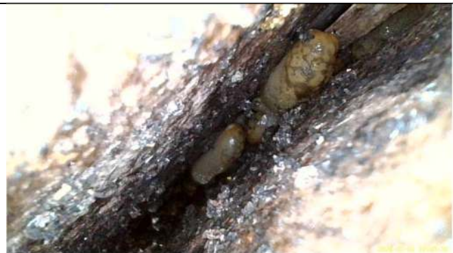
Photograph 10. Endoscopic view of the sheer crack in one of the trees in tree group G2
