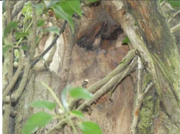
Photograph 12. Close-up of branch drop in one of the trees in tree group G2
