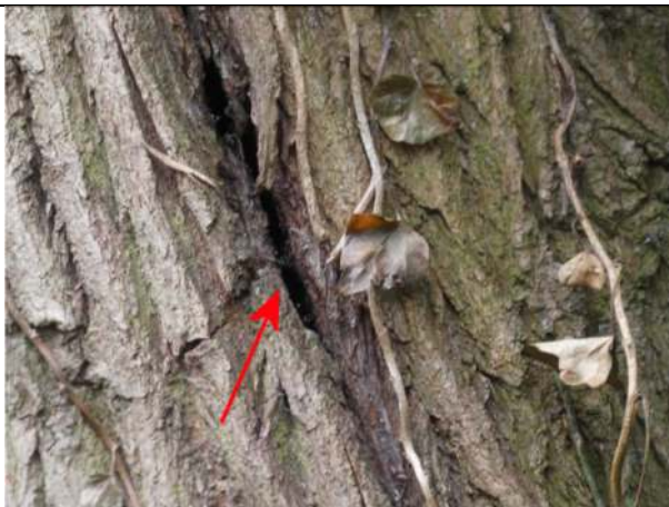
Photograph 9. Sheer crack in one of the trees in tree group G2
