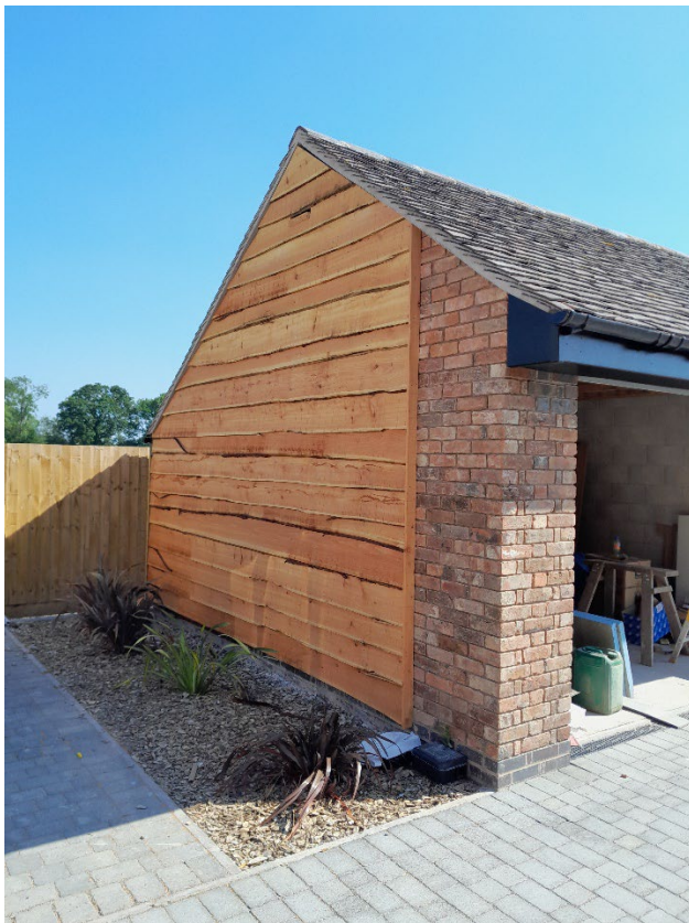
Fully clad western elevation.
