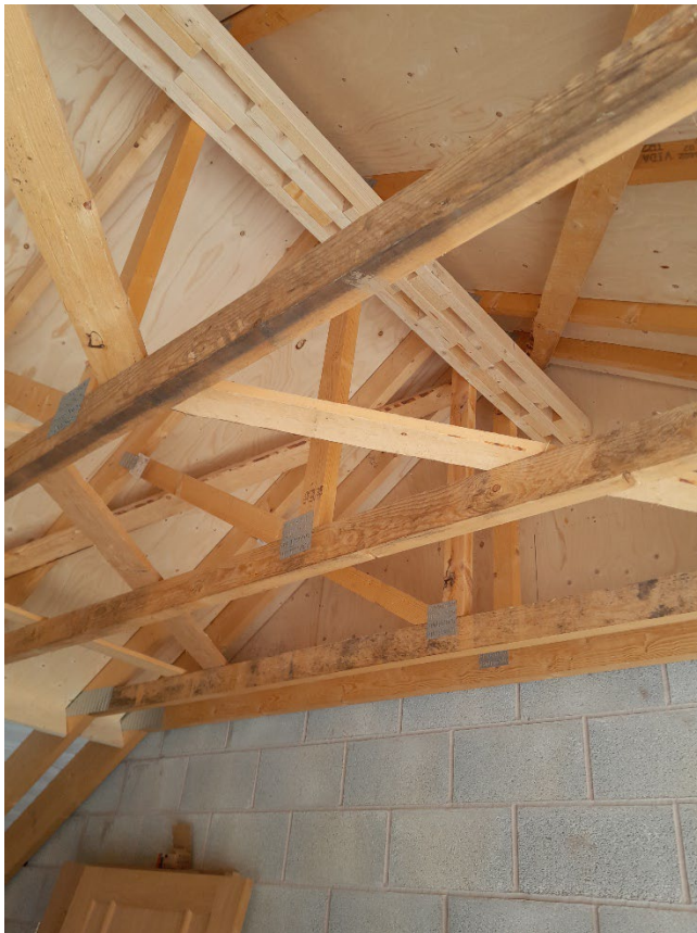
Crevices created in timber within western roof space after all bat loft lined with plywood.
