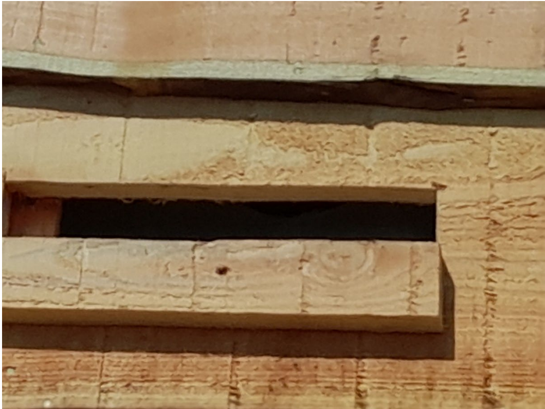
Core drilled hole just visible above access on eastern elevation.
