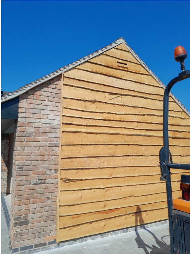
Fully clad eastern elevation.
