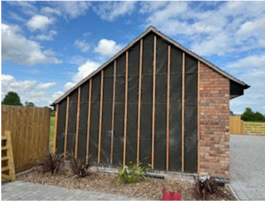
Bitumous underfelt installed on western elevation.
