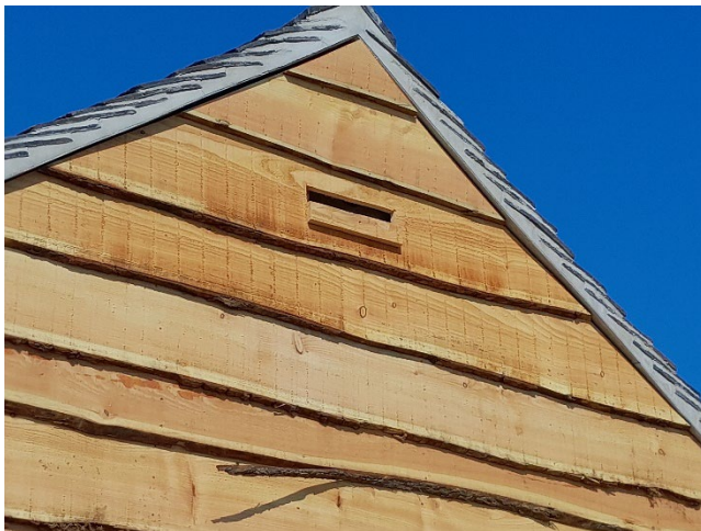
Bat access with platform and access to rear of waney edge cladding.
