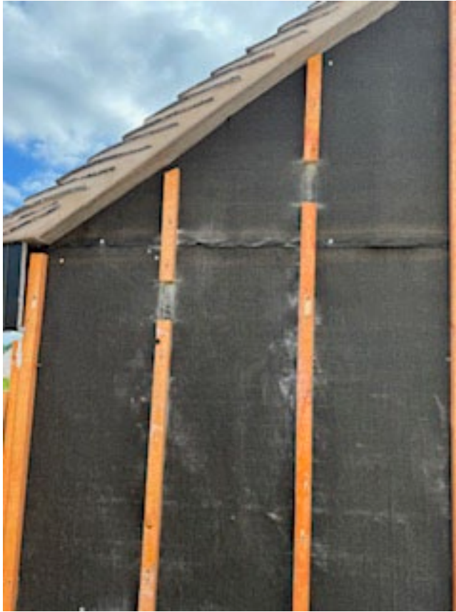
Gaps cut in timber battens on eastern elevation.
