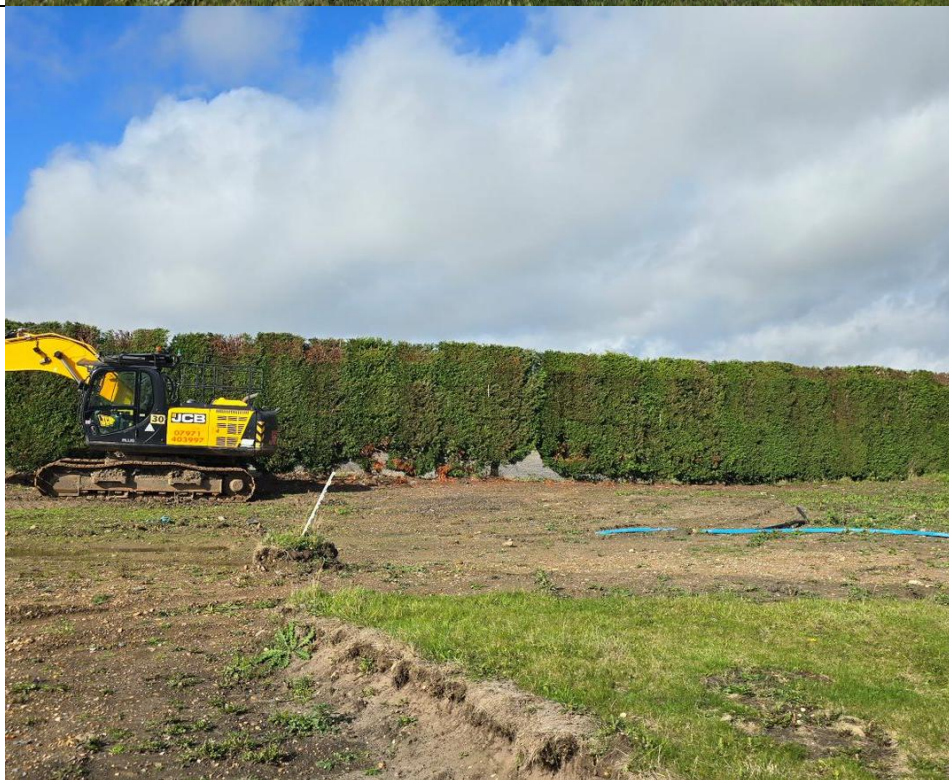
Plate 6: Image showing the site clearance and line of trees.
